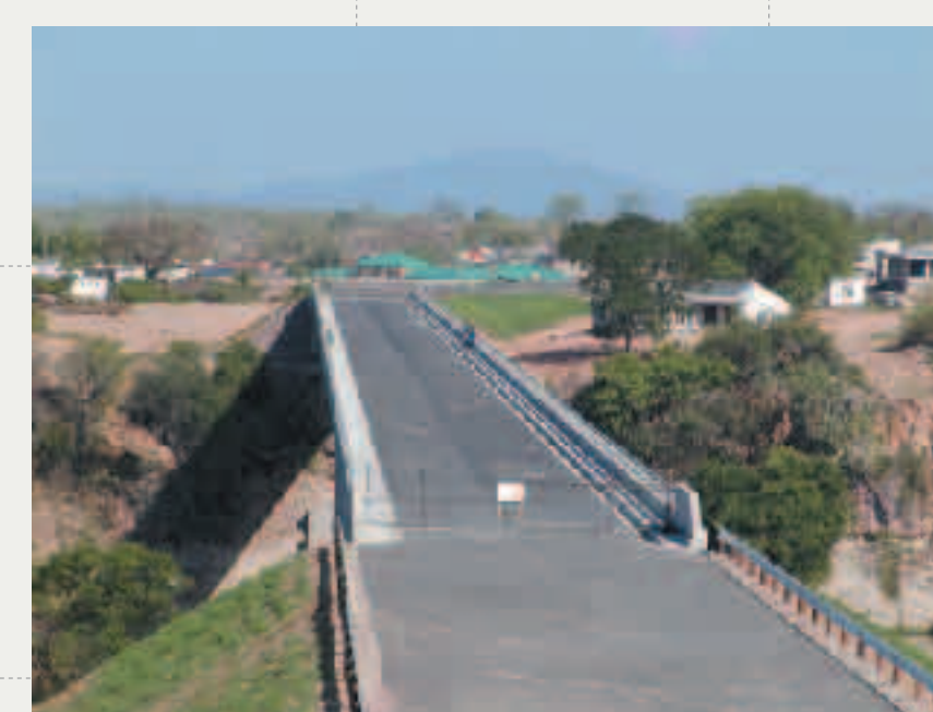
New Bridge over the Zambezi River at Chirundu Border Post (between Republic of Zambia and Republic of Zimbabwe) (Grant Aid 1998-2002)
