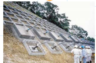
Slope Protection using concrete frame slope protection.
