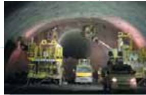
Shimizu No. 1 Tunnel: Enlargement of excavation area by NATM
