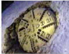
Shimizu No. 1 Tunnel: TBM
