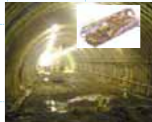
Shimizu No. 4 Tunnel
