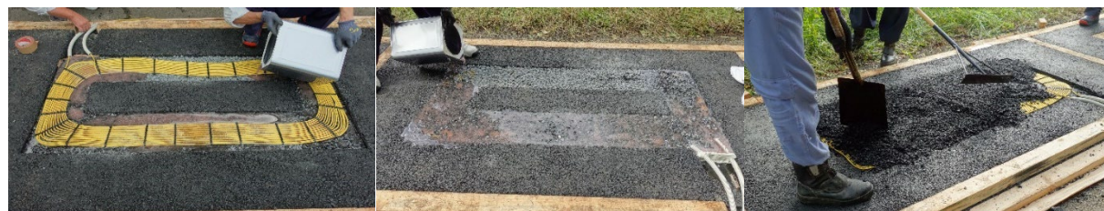
(a)樹脂20 mm (b)樹脂40 mm (c)直接埋設
