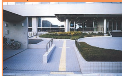
視覚障害者誘導用床材の敷設 緩やかな勾配の手すり付きスロープ Tactile ground surface indications installed on floor Gentle slope with handrails
