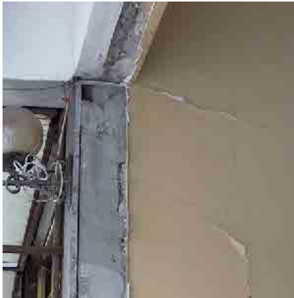
1) Mortar does not fall down, and only small cracks are observed on mortar.
