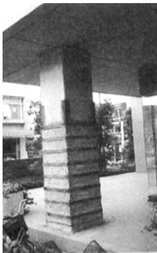
(6) Jacketing of damaged column with steel sections [1]
