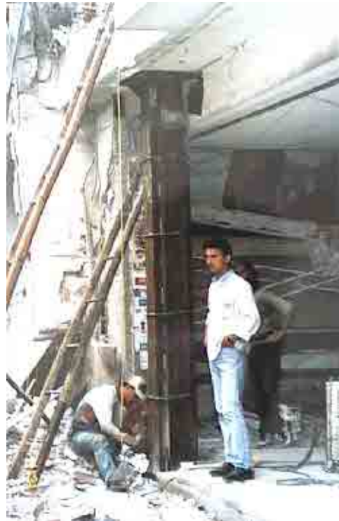
(9) Shoring with steel sections beside a column damaged due to pounding (left: before retrofit, right: after retrofit)
