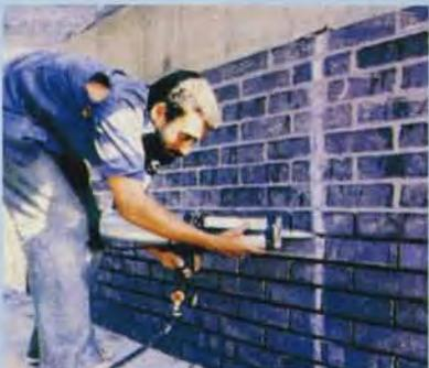
*Lining culvert with acid-resistant blue bricks*
