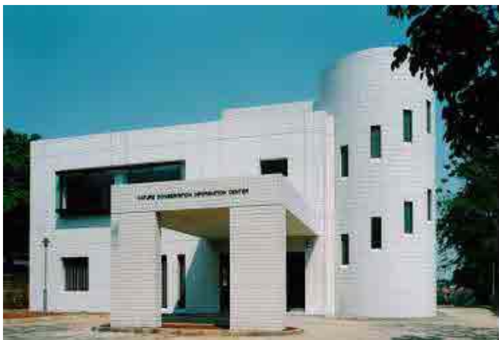
Picture 1 The exterior appearance of the NCIC
