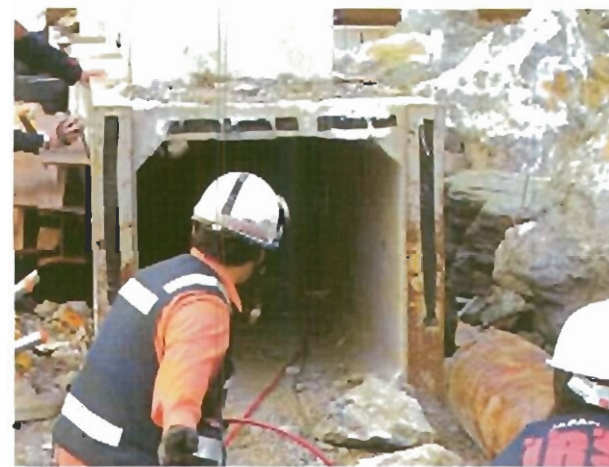
(4) Cutter Robot cut reinforcing bar.
