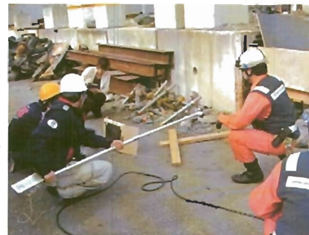
(3) Multi-sensor head measured shape of the hole and obstacles.
