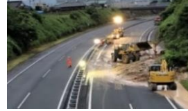
Use two non-affected lanes to ensure transportation function
