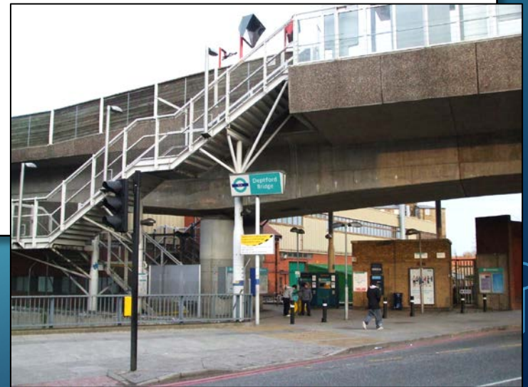
Deptford Bridge Station (Docklands Light Railway : GB)
