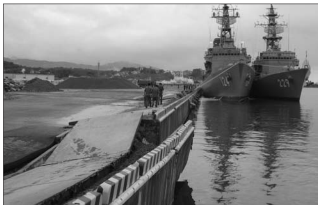
●網走港防波堤の被災(冬期風浪)
