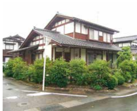
Roof range with beautiful roof tiles (Yatsuo, Toyama Prefecture)
