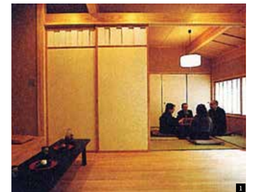
Interior doors which incorporate muso (window made of narrow boards connected on two rails each of which slides for opening and closing) on the top for interior ventilation
