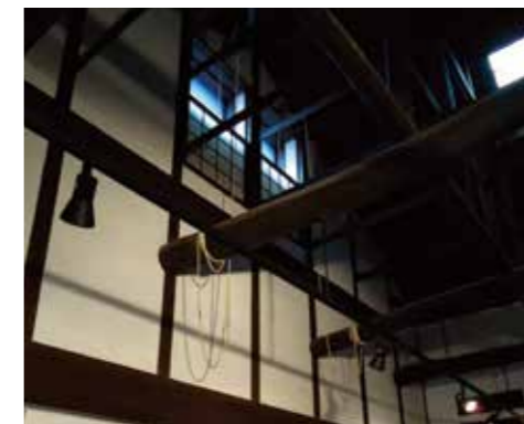
High windows and skylight provide lighting and ventilation for earthen floor rooms in a traditional townhouse
