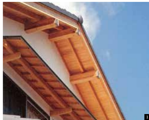
Window eave mounted above window on the gable side
