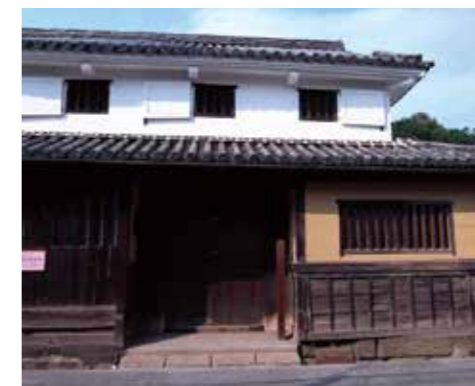
Plaster coated wall of a traditional Japanese house
