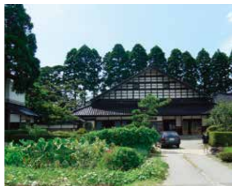
Azuma-dachi is a local way of building houses which face the east from which gentler winds blow. On the west side, vegetation called kainyo is planted. (Toyama Prefecture)
