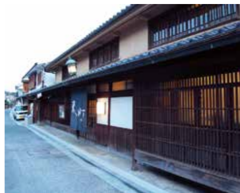
In this traditional townhouse, the lattice was set to keep people outside from seeing in.
