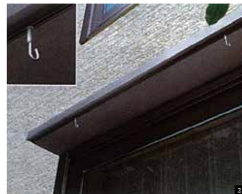
Hooks attached underneath the eaves to hang sunscreens.
