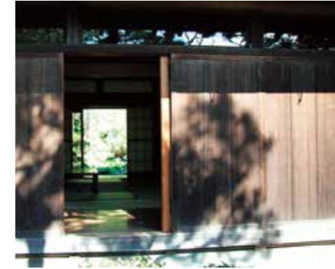
Wooden sliding storm doors of a typical traditional house
