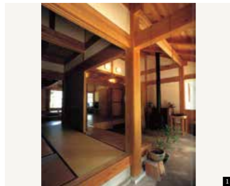
The central pillar stands between doma earthen floor and zashiki rooms. The door sills were originally designed slightly outward which required to cut the corner of the tatami mat to give a space for the central pillar. To avoid this, the door sills were moved inwards to match the inside corner of the central pillar.
