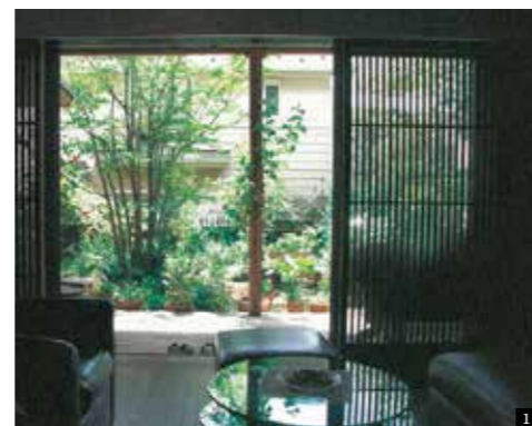
When lattice doors are closed, one can see from inside but cannot be seen from outside, while allowing ventilation and cutting glare of sunshine.
