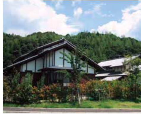
Sloped roofs quickly drain off the rain to make roofs more resistant to rainwater. (Oita Prefecture)
