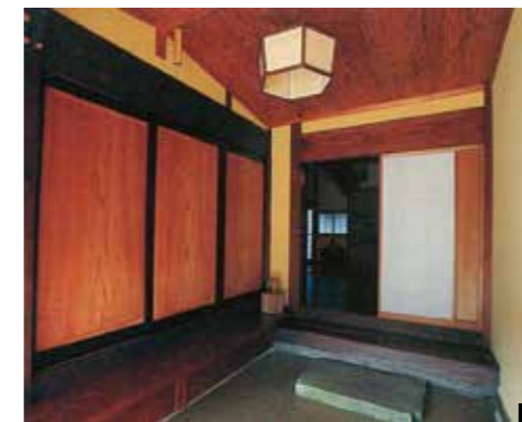
Wood board sliding doors for partition in a traditional house
