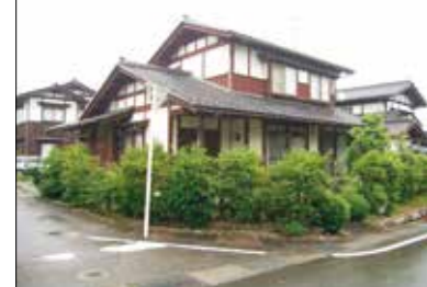
Sloped roof with tiles (Toyama Prefecture)
