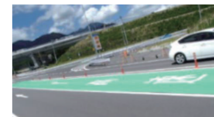
Measures at the entrance and exit of expressways (Colored pavement)
