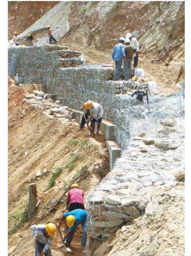
ガビオン(布団かご) 擁壁 / Gabion (cage filled with stones) retaining wall
