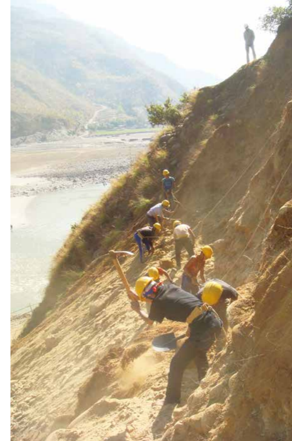
重機投入が難しい場所の人力掘削 / Manual excavation in a location difficult to access by heavy machinery
