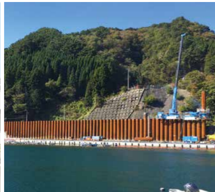
防潮堤の災害復旧工事(岩手県) / Disaster recovery work on seawalls (Iwate Prefecture)
