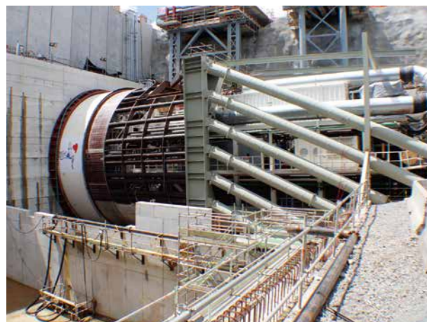
1本目トンネル、発進前の坑口付近の状況/ Scene near the entrance of the first tunnel prior to launch
