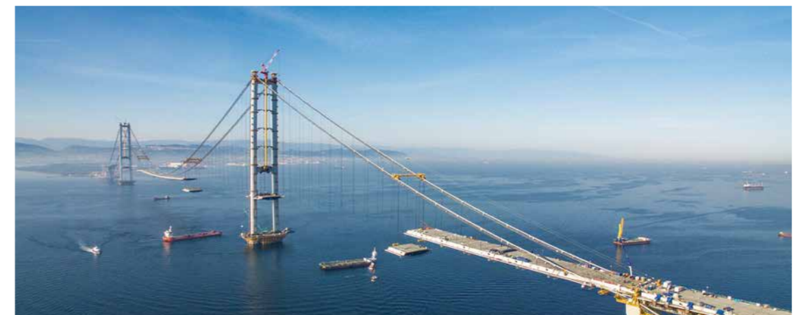
補剛桁架設／Erection of main deck segments
