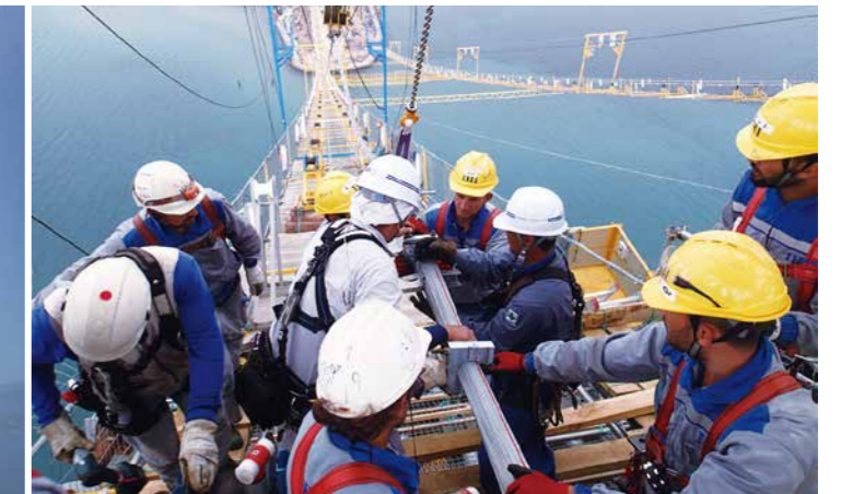
南側主塔塔頂でのケーブル架設作業。日本人橋梁特殊工とトルコ人ワーカーとの共同作業／ Cable installation work at the top of the south main tower. Collaboration between Japanese supervisors and Turkish workers
