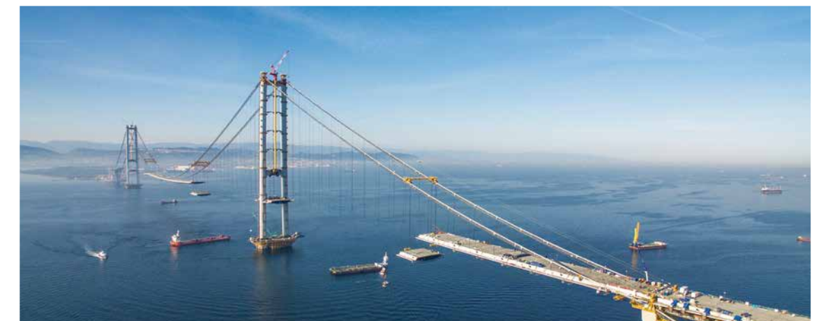
補剛桁架設／Erection of main deck segments
