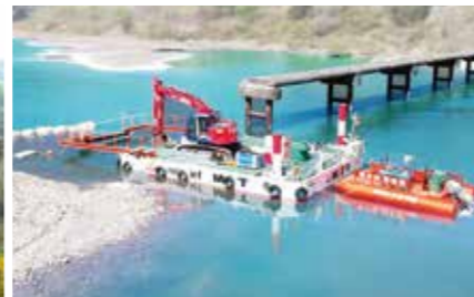
組立式台船災害復旧工事 (高知県) / Disaster recovery for assembled barges (Kochi Prefecture)
