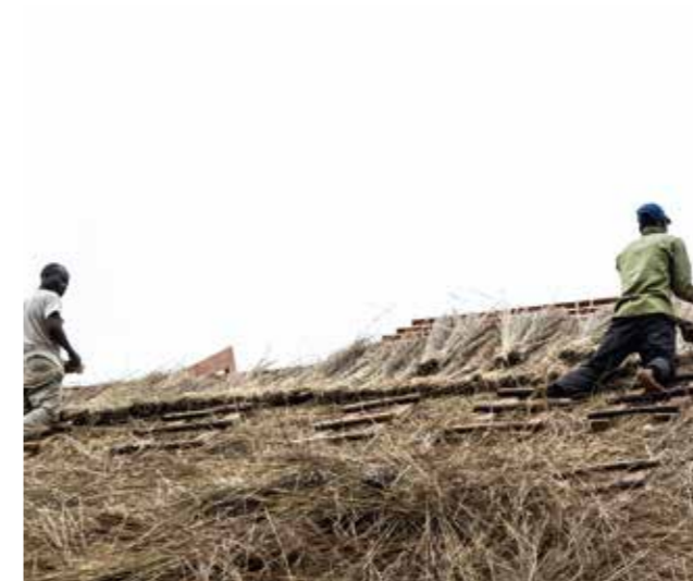
茅で屋根を葺く職人たち／ Craftspersons covering the roof with thatch
