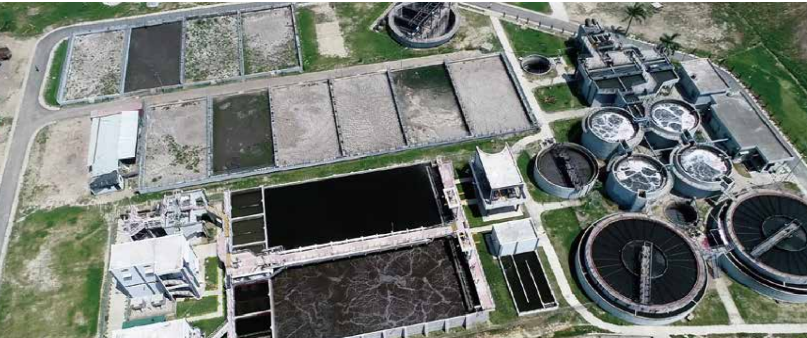
サロリ下水処理場全景(既設含む) / Salori Sewage Treatment Plant (overall view including existing facilities)
