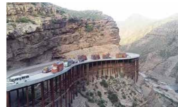
パキスタン国道 N70号改修工事 SqCピア工法本橋区間 / Repair of Pakistan National Highway N70; application of SqC pier method to final bridge section
