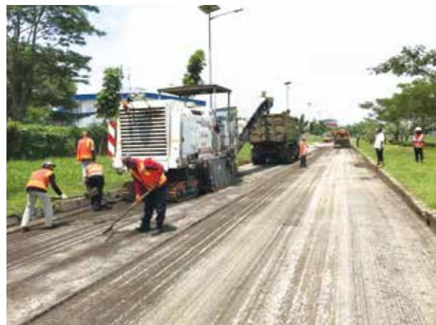
工業団地内の路面切削状況 / Road surface cutting work in industrial park
