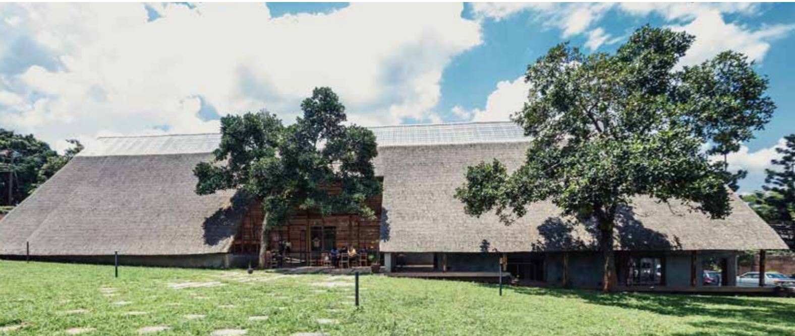
東側からの立面。敷地のスロープと既存の樹木を生かした／ View of the facility from the east. The design makes the most of the slope of the site and the existing trees
