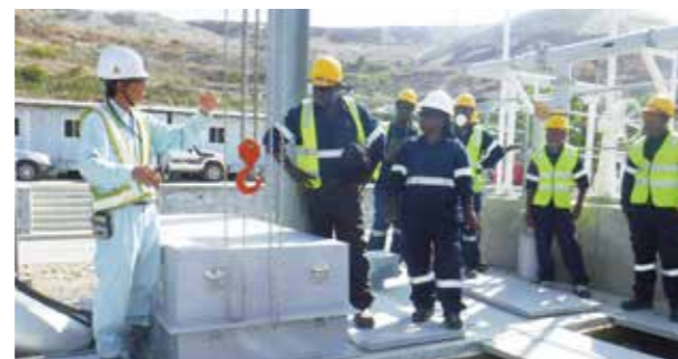
下水処理機器メンテナンス指導状況/ Instruction on the maintenance of sewage water treatment equipment
