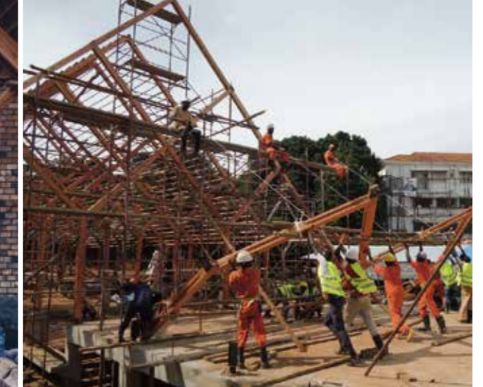
重機を使わず人力で地組したフレームを立ち上げる／ Manually erecting the framework that had been assembled on the ground, without the use of heavy machinery
