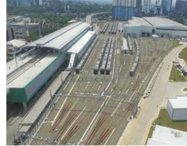
日本の車両基地をモデルに設計・施工したレバックブルス車両基地／ Lebak Bulus Depot was designed and constructed based on Japanese depot models
