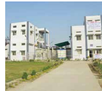
電気設備棟と管理・水質検査棟 / Building of electrical equipment and building of administration and water quality inspection
