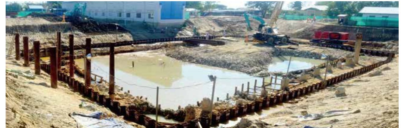
ミャンマーニャウフナッピン浄水場基礎工事 / Foundation construction for Nyaungnaping Water Treatment Plant in Myanmar
