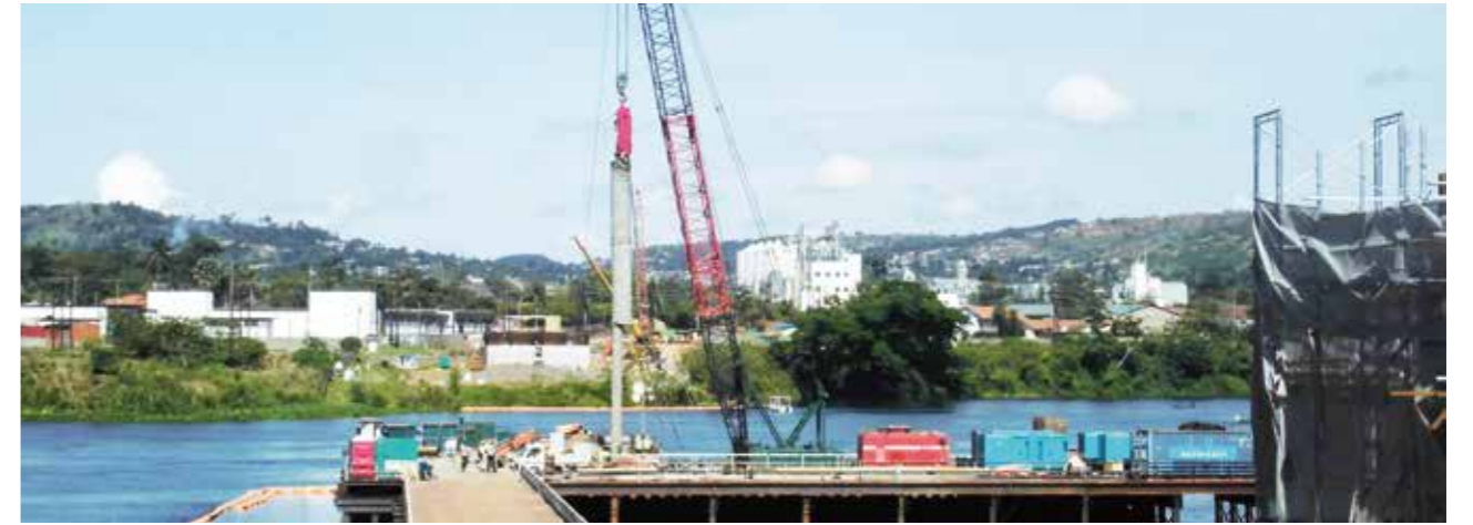
ウガンダナイル川斜張橋基礎工事 / Foundation construction for cable-stayed bridge across the Nile in Uganda
