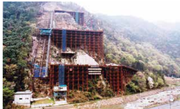
広島空港大橋 仮栈橋・構台工事(広島県) / Construction of temporary piers and assembly base for the Hiroshima Airport Bridge (Hiroshima Prefecture)
