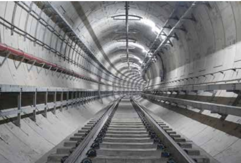
漏水の無い高品質のトンネルがインドネシアで初めて完成／ Tunnel of high quality without leakage was completed in Indonesia for the first time
