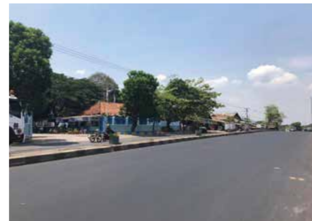
西ジャワ州道の試験施工/ After test application to road in West Java
