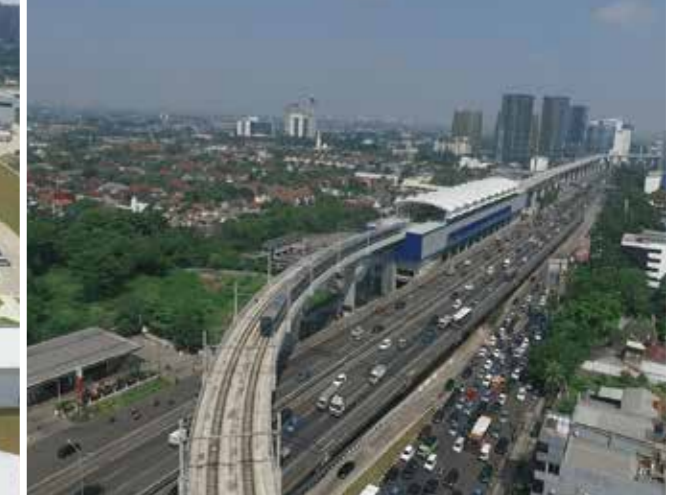
ファトマワティ駅と高速道路を跨ぐ急曲線長大橋／ Long span bridge with small radius curve over toll road near Fatmawati Station
