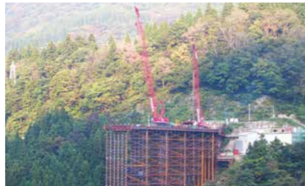
利賀ダム 仮栈橋工事(富山県) / Construction of temporary piers for the Toga Dam (Toyama Prefecture)
