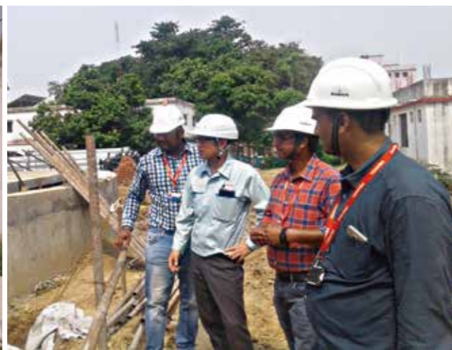
ガンジス川浄化計画に継続参画、ビハール州の下水処理場での日本人技術者による指導の様子。 Ongoing participation in the Ganges purification plan. A Japanese engineer providing guidance at a sewage treatment plant in the State of Bihar
