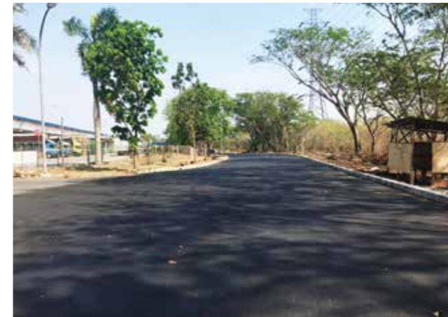
工業団地内の施工後/ After application in industrial park
