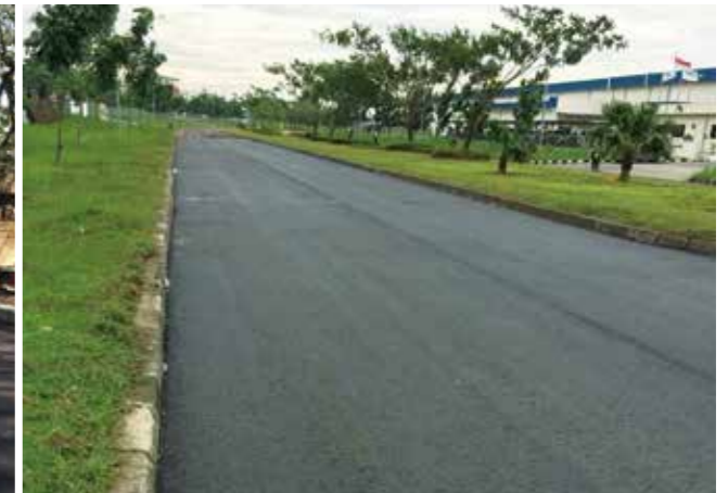
工業団地内の試験施工後/ After test application in industrial park
