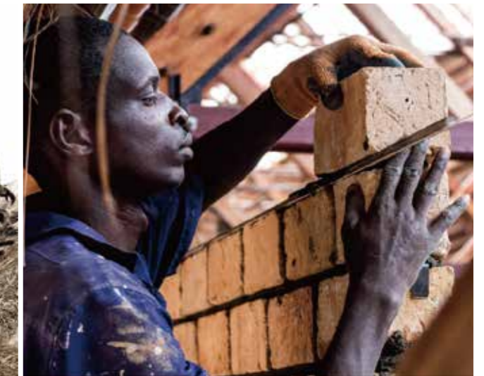
現地で最も汎用性のある焼成レンガを丁寧に積んでいく／ Carefully stacking fired bricks, one of the most versatile materials in the area
