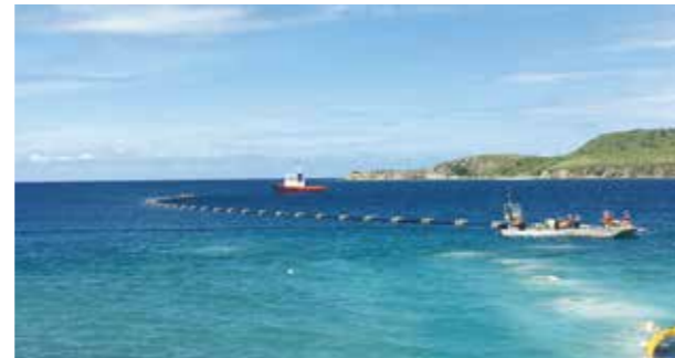
海中放流管施工状況/Installation of an ocean outfall pipe
