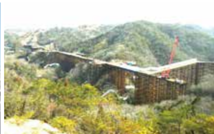
SqCピア工法 鋼管橋脚工事 (兵庫県) / Steel pipe pier construction using the SqC pier method (Hyogo Prefecture)
