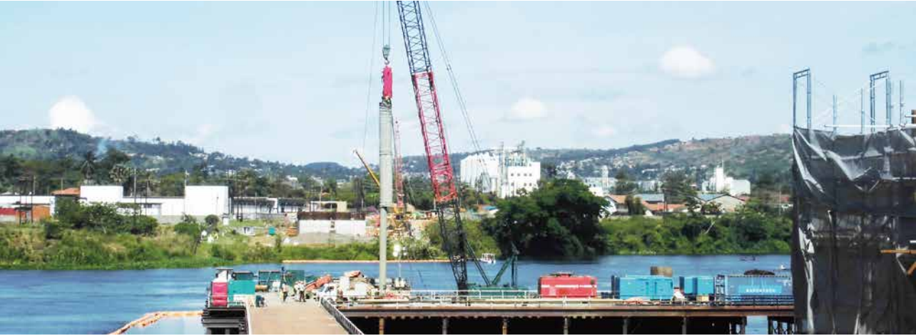
ウガンダナイル川斜張橋基礎工事／Foundation construction for cable-stayed bridge across the Nile in Uganda
