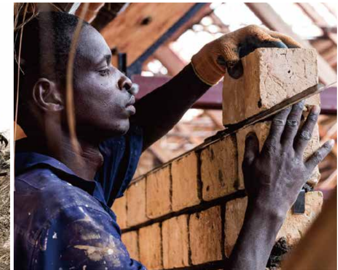
現地で最も汎用性のある焼成レンガを丁寧に積んでいく／ Carefully stacking fired bricks, one of the most versatile materials in the area
