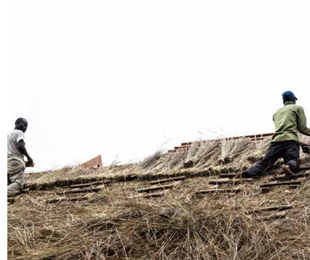
茅で屋根を葺く職人たち／ Craftspersons covering the roof with thatch
