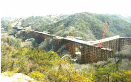
SqCピア工法 鋼管栈橋工事（兵庫県）／ Steel pipe pier construction using the SqC pier method (Hyogo Prefecture)
