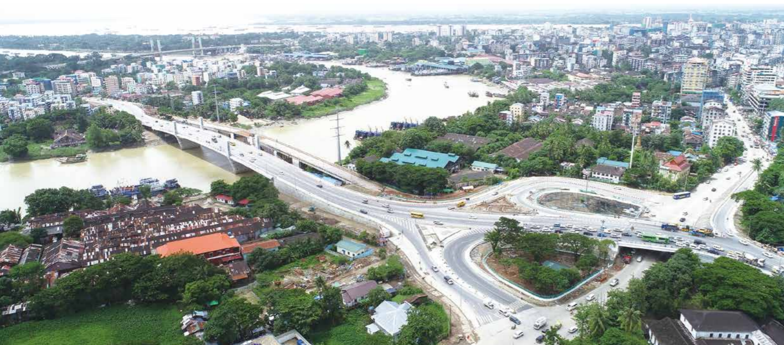
新タケタ橋のプロジェクト全景／Overview of the project for the construction of New Thaketa Bridge
