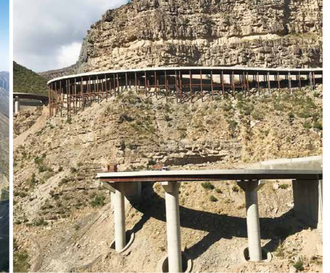
上: 鋼製床版拡幅橋梁、下: 鋼製箱桁橋梁 / Upper: Pre-fabricated steel widening bridge; Lower: Steel box girder bridge
