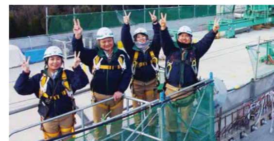
1期生のダニー(一番左)、九州のPC橋上部工現場にて／ Dany (leftmost), a member of the inaugural class, on a PC bridge superstructure site in Kyushu
