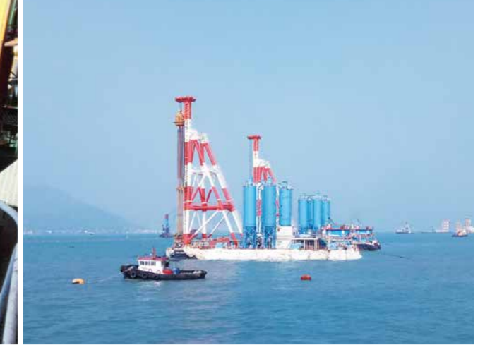
CDM改良船とシルトフェンス(二次バリア) / CDM improvement vessels and silt fences (secondary barrier)
