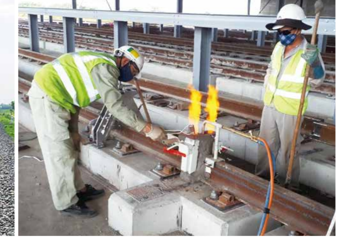
レール溶接技術を習得した協力会社技術者(ベトナム) / Partner company's engineers who acquired rail-welding expertise (Vietnam)
