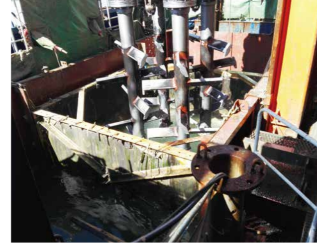
CDM改良機と汚濁防止柵(一次バリア) / CDM improvement device and pollution control frame (primary barrier)
