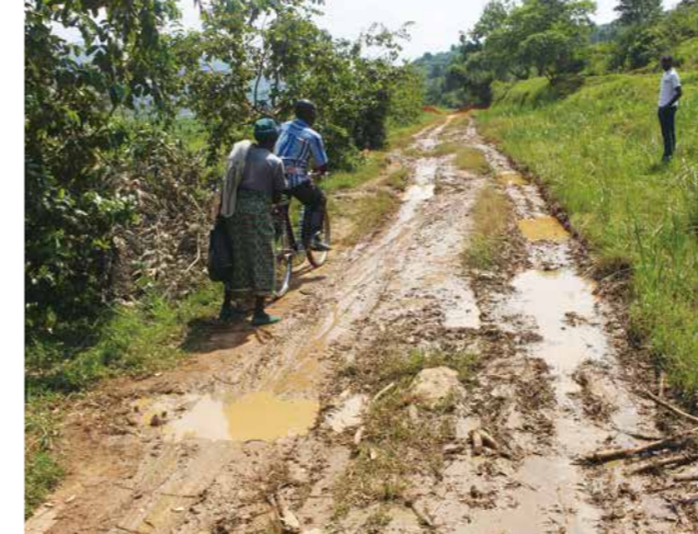
施工前の自転車の走行もままならない道路(ルワンダ) / Road before repair where passing with bicycle is difficult (Rwanda)
