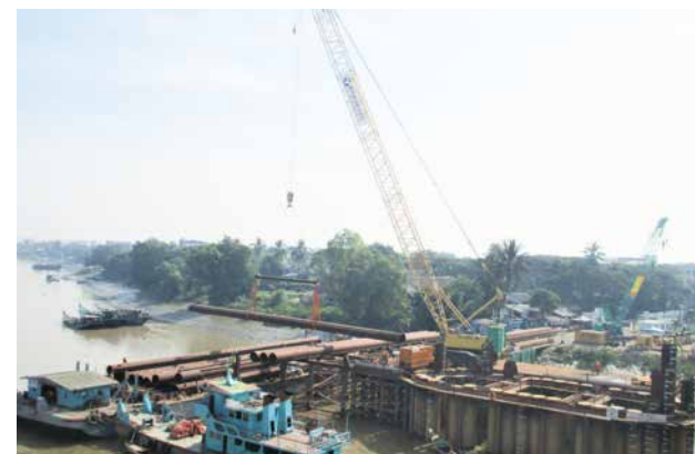
鋼管矢板の搬入と打設工事／ Delivery of steel pipe sheet piles and concrete placement
