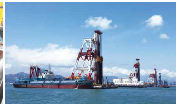
CDM改良船団による地盤改良施工状況／ Work being performed by fleet of CDM improvement vessels
