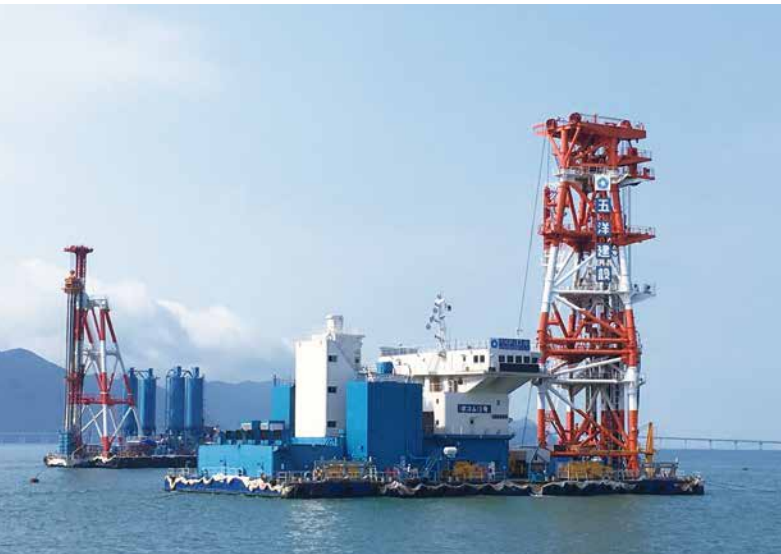
CDM改良船による大規模地盤改良工事／ Large-scale ground improvement work by CDM improvement vessels
