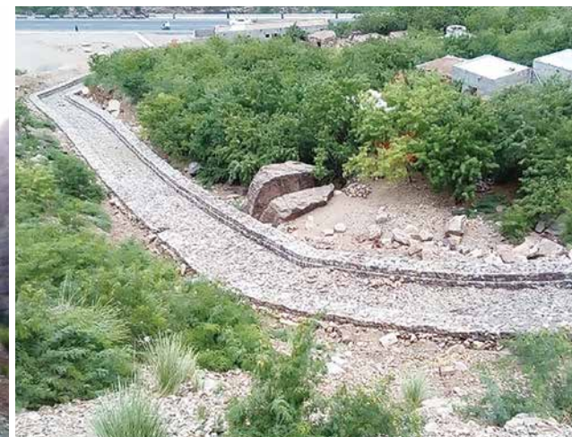
現地石材を用いた排水路／ Drainage canal using locally quarried building stone
