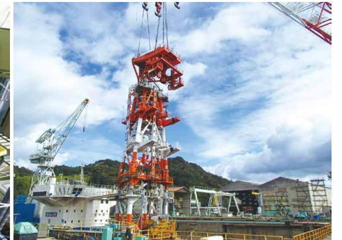
空頭制限対応のための櫓の低頭改造状況／ Lowered scaffold developed in response to overhead space restrictions
