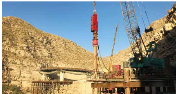
硬質岩盤への鋼管杭打設状況／Steel pipe driven into hard bedrock
