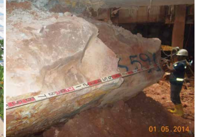
ベンクーレン駅掘削時に出現した巨大転石／ Gigantic boulders that emerged during the excavation work in Bencoolen Station
