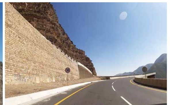
既設の石積み擁壁を有効活用した道路改良（建設後）／Road improvement making effective use of existing masonry retaining walls (after the construction work)
