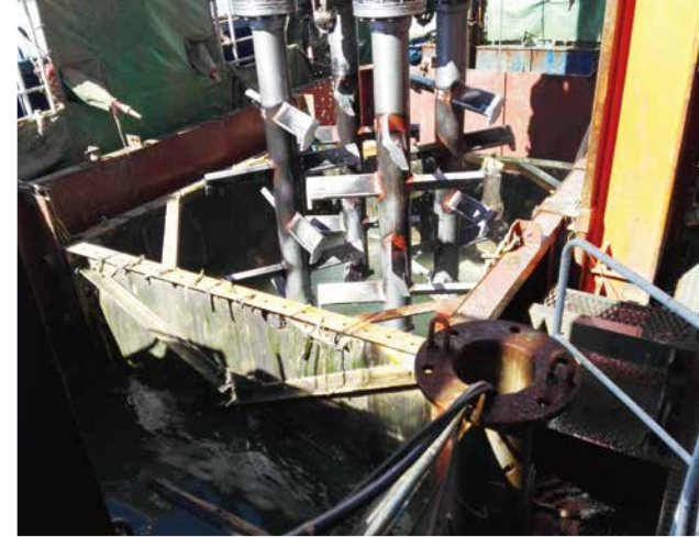
CDM改良機と汚濁防止枠(一次バリア)／ CDM improvement device and pollution control frame (primary barrier)
