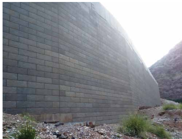
気泡混合軽量盛土工法／ Foamed cement banking method
