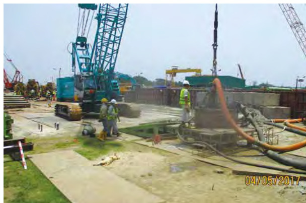
清水を用いた場所打ち杭の施工状況／ Construction situation of Cast in-situ Pile using fresh water
