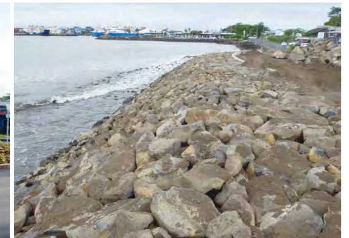
巨石を利用した海岸護岸 (施工中) ／ Seawall built with large rocks (under construction)
