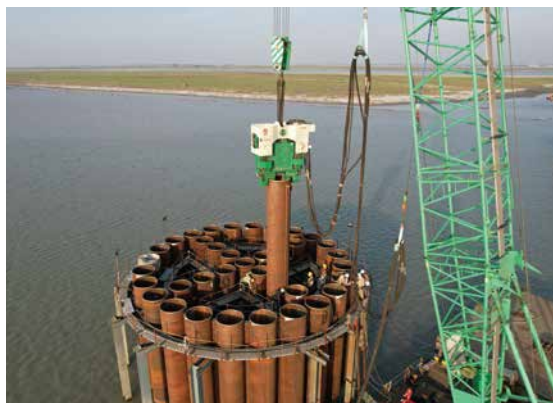
バングラデシュ国バンガバンドゥ鉄道橋基礎の鋼管矢板井筒施工状況／ Construction of a foundation for Bangabandhu Railway Bridge in Bangladesh, using the steel pipe sheet pile well foundation method
