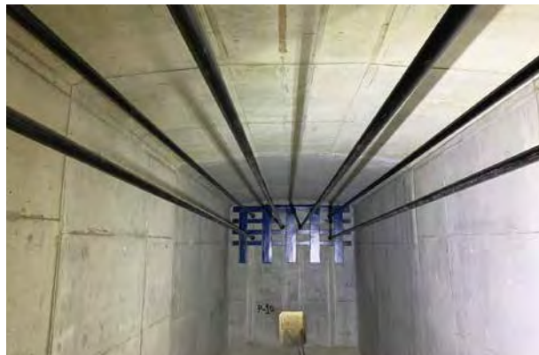
PC外ケーブルを設置・緊張後の既存橋内部／ Interior of existing bridge after installation and tensioning of PC outer cable
