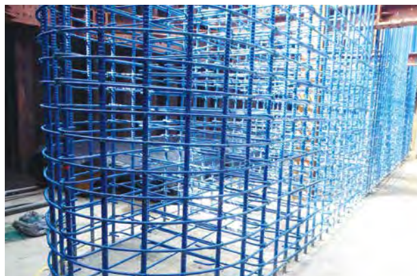
エポキシ樹脂塗装鉄筋を用いた橋脚部／ Bridge piers with epoxy-coated reinforcing steel bars
