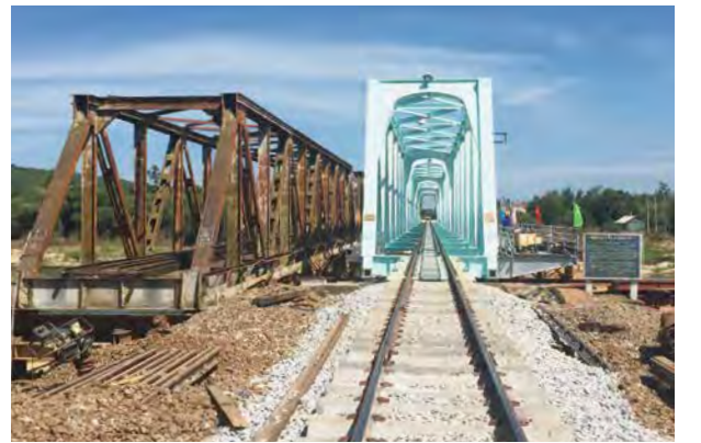
横取り方式で架替えが完了／ The replacement of the bridge is completed using the lateral transfer method
