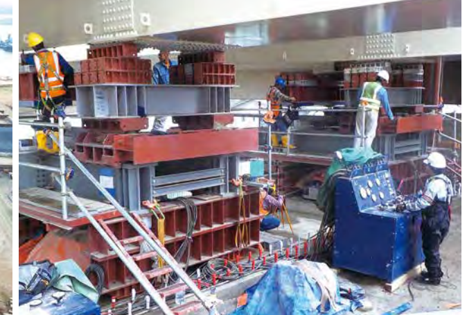
鋼細幅箱桁と合成床版及び送り出し工法の採用／ Adoption of Steel narrow box girder, Steel concrete composite deck slab and Launching erection method
