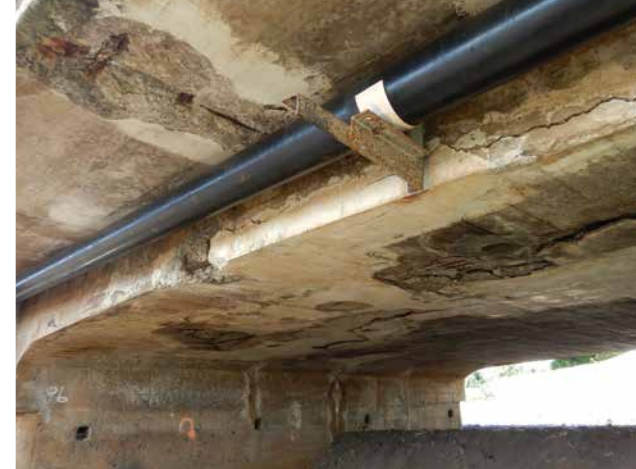
既設橋下面部の劣化状況／ Salt damage to the undersurface of the old bridge
