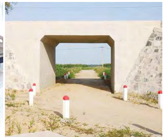
鉄道盛土で分断されている区間には、適所に洪水時の通水を兼ねたアンダーパスを整備／ Underpasses were constructed at appropriate locations along the section divided by the railway embankment to ensure passage for residents and water flow during flooding
