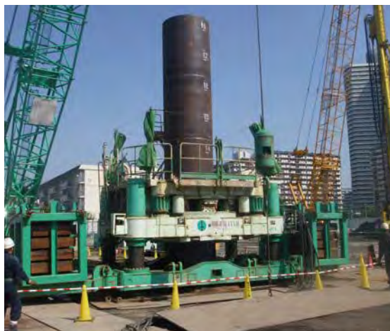
鋼管回転杭施工状況／ Construction work with steel pipe rotating piles
