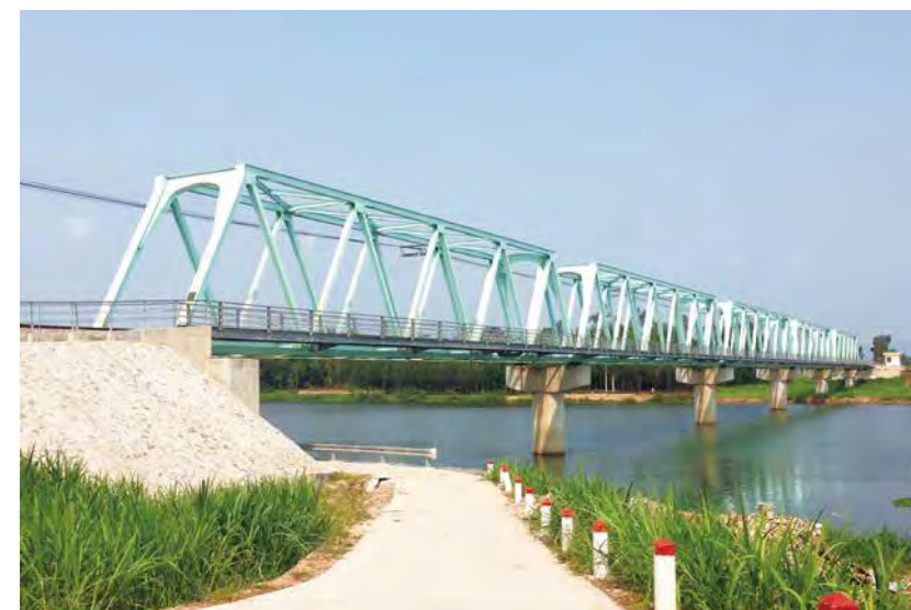
横取り方式で架替えを実施した5径間トラス橋のチャーボン橋／ Tra Bong Bridge, a 5 span truss bridge that was replaced using the lateral transfer method
