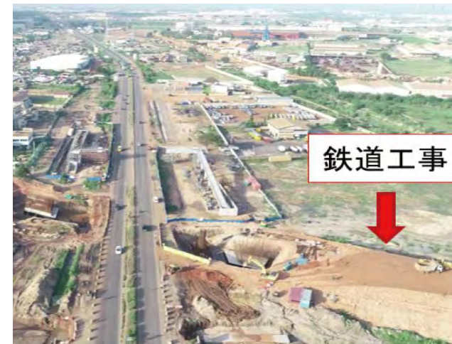
ドローンの活用例：鉄道工事との干渉状況を関係者に視覚的に認知してもらうことで早期解決を実現／ Example of use of drones: Realization of early resolution by having concerned parties visually recognize the situation of interference with railway construction
