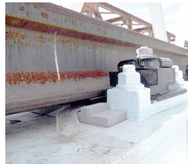
桁設置精度が軌道精度に直結する鋼直結軌道／ Direct fastening system where girder installation accuracy is directly related to track accuracy
