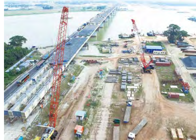
鋼細幅箱桁と合成床版及び送り出し工法の採用／ Adoption of Steel narrow box girder, Steel concrete composite deck slab and Launching erection method
