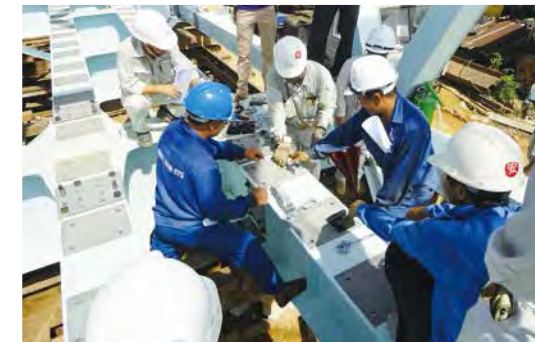
レール締結装置の取付け講習会の様子(各橋梁にて実施)／ Rail fastening device installation workshop (conducted at each bridge)
