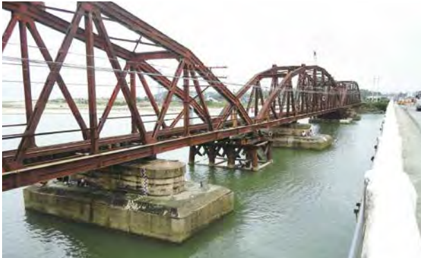
仮復旧状態で運行中の橋梁（鋼製橋脚の腐食が著しい）／ Bridge in operation under temporary restoration status (steel piers are severely corroded)
