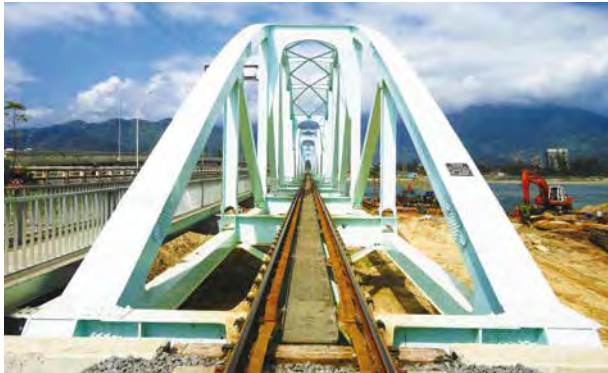
枕木を省略した軌道構造で橋梁高を抑え鋼材使用量を抑制／ Track structure without sleepers to reduce bridge height and steel usage
