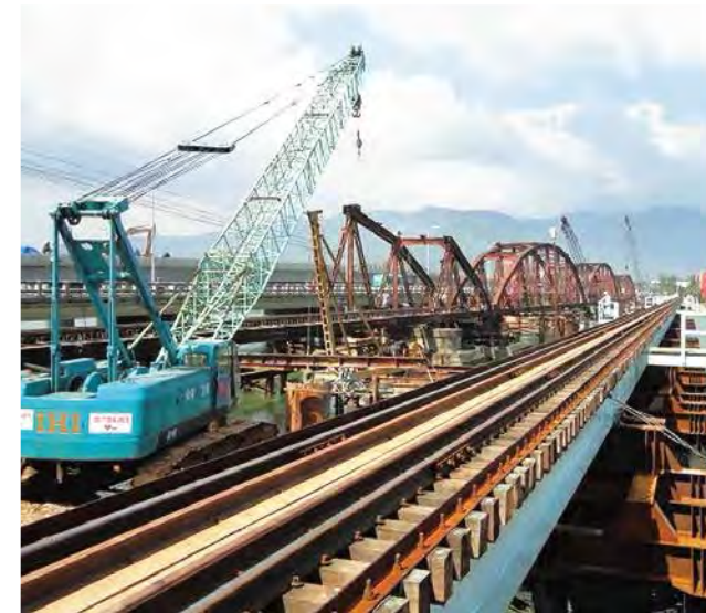
橋梁前後で線形をシフトして仮線で運行を確保し、橋梁改修作業を実施中のNam O橋／ Nam O Bridge undergoing bridge rehabilitation work by shifting the alignment before and after the bridge and securing operations with temporary lines
