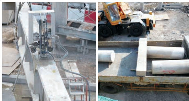
旧橋（取付橋）をブロックに切断し場外へ搬出した／ The old bridge (approach bridge) was cut into blocks and transported outside the site.
