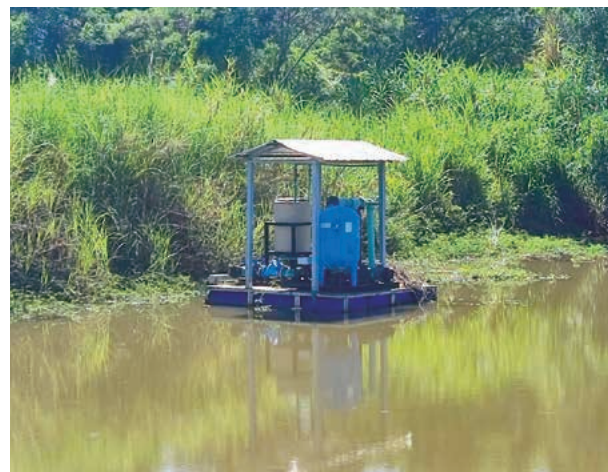
拡張工事で新設した貯水池から貯水槽に水を送るポンプ／ Pump to send water to the water tank from the reservoir newly created in the expansion work
