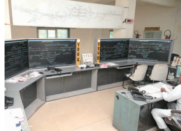
North Western Railway Ajmer駅電子連動装置 制御盤／ Operation console of electronic interlocking system for Ajmer Station, North Western Railway
