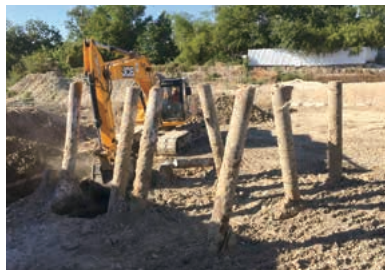
新線橋梁 既設橋梁の斜杭基礎状況／ Route Neuve Bridge: Condition of existing foundation (inclined piles)
