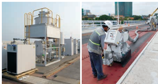
鋼桁・SFRC舗装・鋼製柵等の旧塗装ケレンに採用／ Used for removing old paint from steel girders, SFRC pavement, steel shoe, etc.
