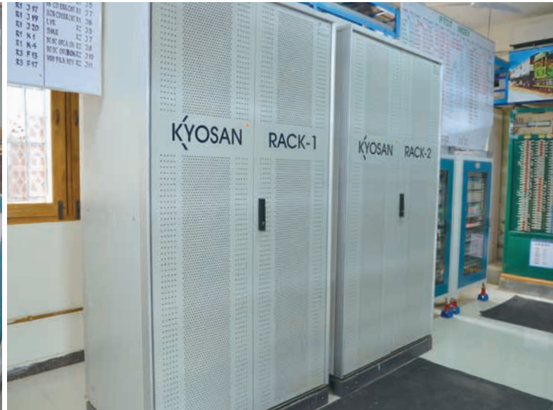
Southern Railway Teni駅電子連動装置 論理端末架／ Logic & Terminal Rack of Electronic Interlocking System for Teni Station, Southern Railway
