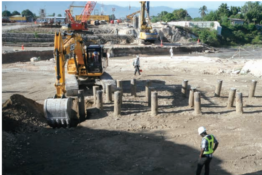
新線橋梁 既設橋梁の杭基礎状況／ Croix-des-Missions Bridge: Condition of existing foundation
