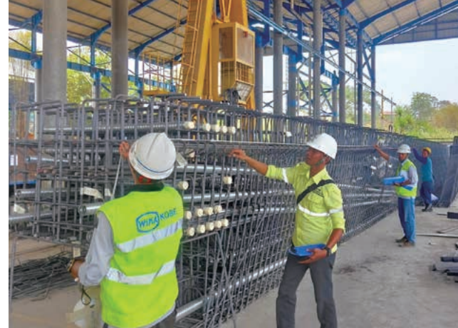
プレキャストU字断面図桁の製作／ Creation of precast concrete girders having U-shaped cross section
