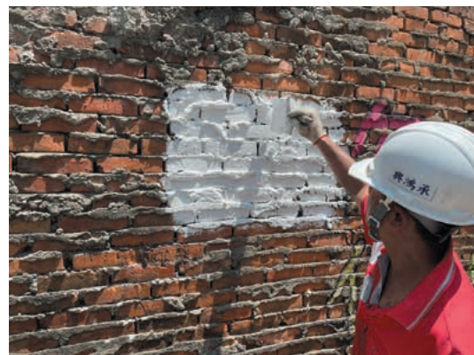
台北の築40年以上のレンガ外壁に施工中。目地の空隙にも充填して連結／Construction in progress on a brick exterior wall in Taipei that is over 40 years old. Filling and connecting the joint voids as well.
