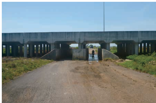
パイルドスラブ構造 (どこでも道路横断が可能) / Piled Slab Structure (allows locals to cross to the other side of the road)
