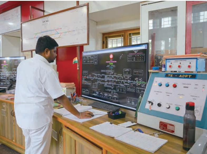
Southern Railway Teni駅電子連動装置 制御盤／ Operation Console of Electronic Interlocking System for Teni Station, Southern Railway
