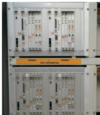
電子論理部。従来型のリレー論理回路に比べ電力削減効果がある／ Electronic logic part that provides power savings compared to the conventional relay logic circuit
