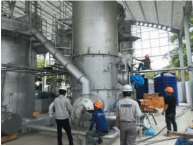
ユニットで輸送、現地組立を実施／ The system is transported as a unit and assembled locally.
