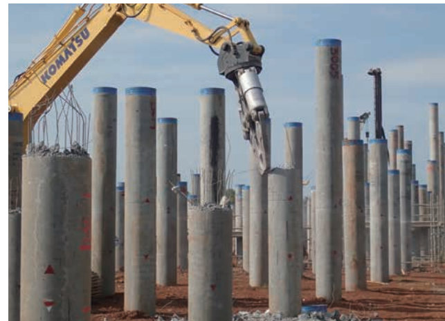
大割機「ガジラ」による杭頭処理／ Pile Head Treatment Using the Large Breaker "Gudzilla"
