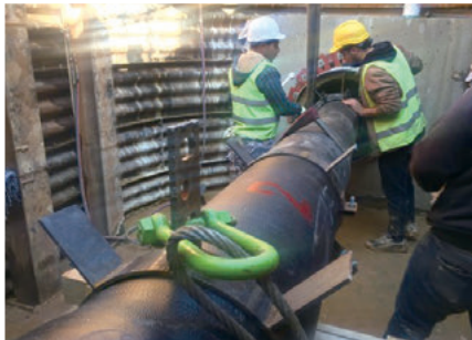
Water Transmission Pipeline Insertion at Pipe Jacking Location
