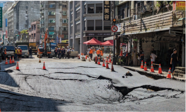
Sinkholes and roadway collapse due to aging infrastructure and natural disaster have become increasingly important issues within Taiwanese society, and in response the government has implemented proactive policies supporting strategic subsurface cavity detection surveys.
