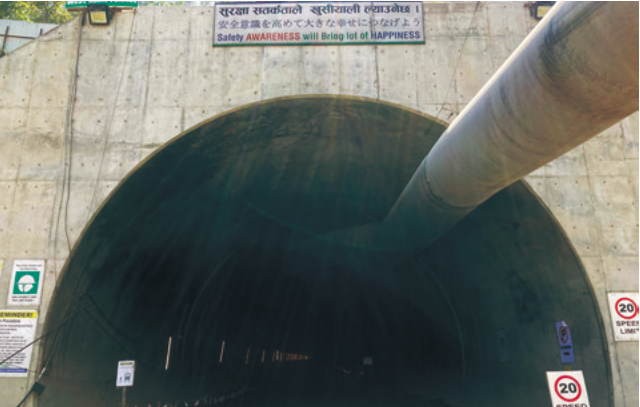
Nagdhunga Tunnel Project where our product was used in the secondary lining concrete
