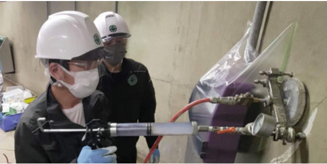
Crack repair was carried out on 0.1mm wide cracks in the walls of Luz Station, São Paulo, Brazil, by injecting self-healing material.
