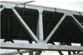
Matadi Bridge under repainting works (The left half has been repainted)
