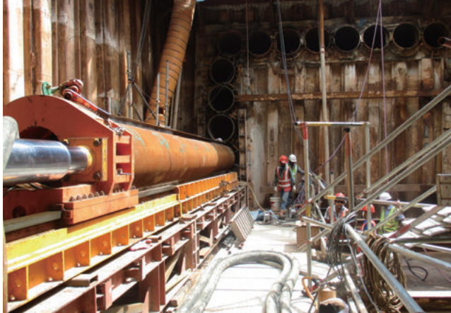
Implementation of the pipe roof method using a Retractable Micro TBM
