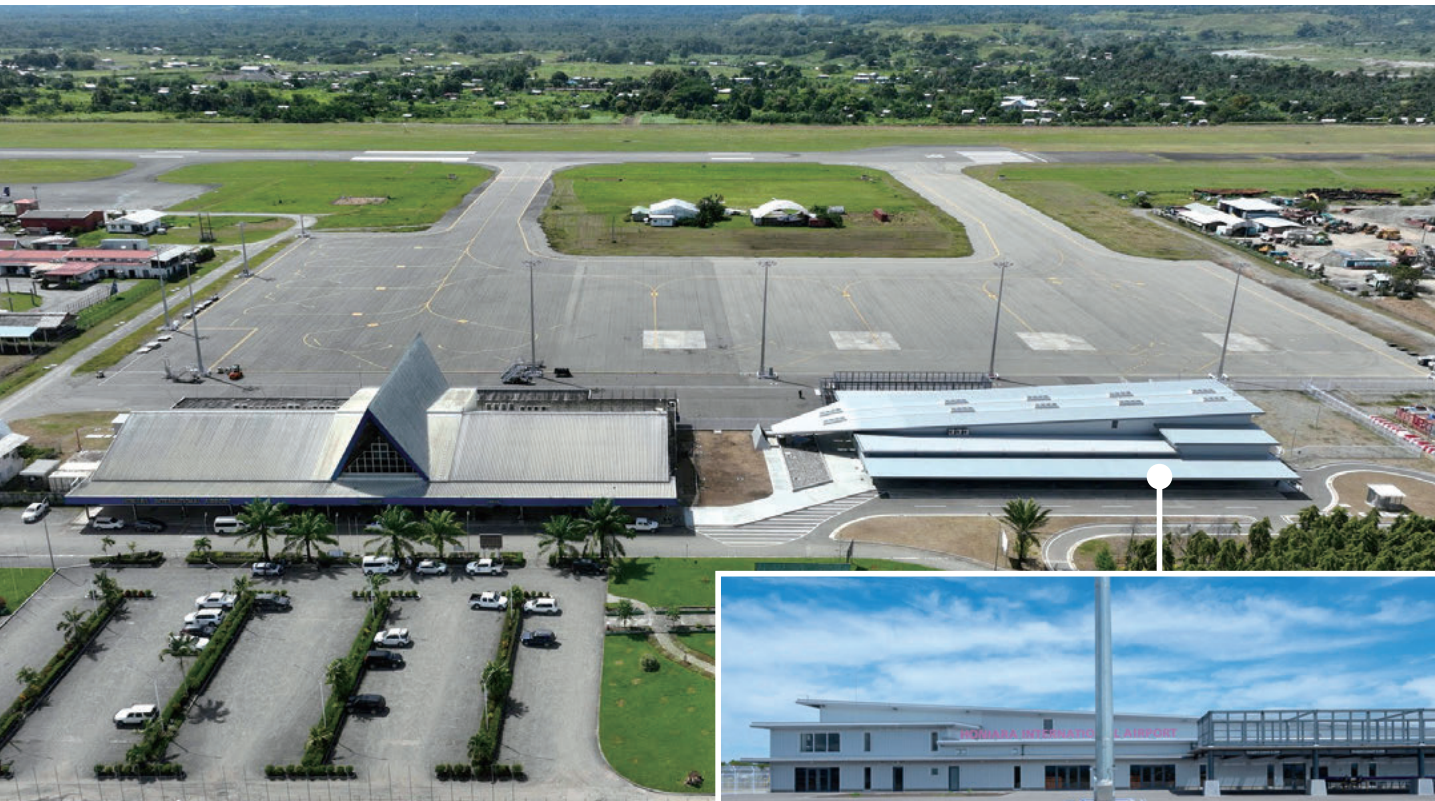
The new international departure terminal building (right bottom), The renovated former international terminal building (left bottom), and the expanded apron (center)
