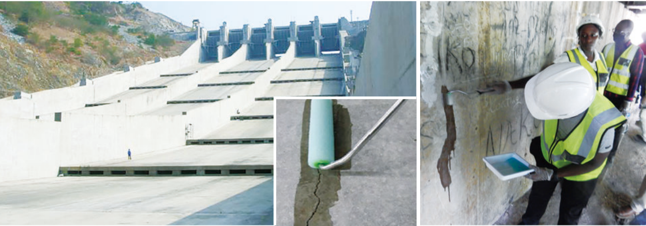
Repairing thousands of meters of cracks in the spillway under construction at San Roque Dam in the Philippines.
