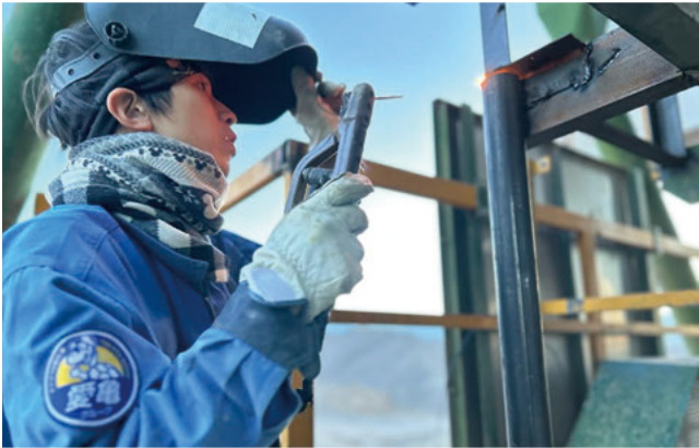
JICA SDGs Business Supporting Survey "Road Maintenance using All-Weather Pavement Repair Materials in Kyrgyzstan". (The asphalt plant modification for manufacturing technology transfer.)
