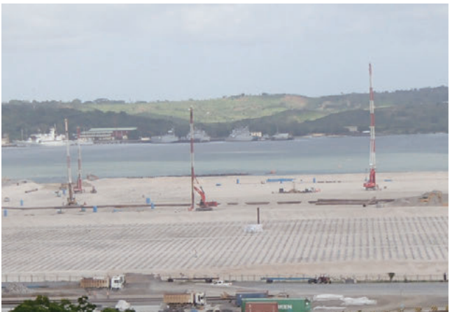
PVD installation in progress: 4.25 million meters of vertical drains were installed in soft clay soil to accelerate consolidation for the container yard
