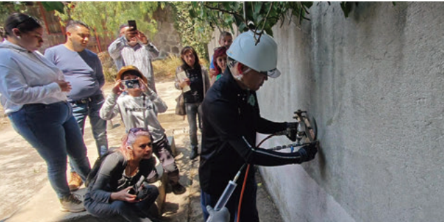
Demonstration of crack injection conducted for Mexico City Government officials.
