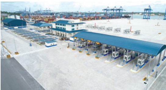
Port Facilities including Administration Complex Building (Center), Container Gate (Right), Welfare Building (Left) and Mechanical Equipment Workshop (Back Left).
