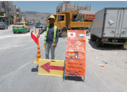
Safety Management at Construction Vehicle Access Points in Urban Pipeline Construction Areas (Arrangement of Traffic Guards)
