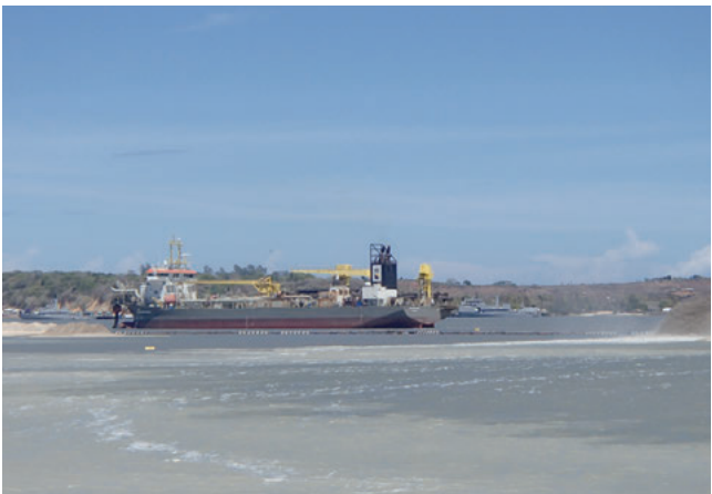
Reclamation by Trailer suction hopper dredger. Rapid land reclamation using 3 million m³ of sand from the Indian Ocean.
