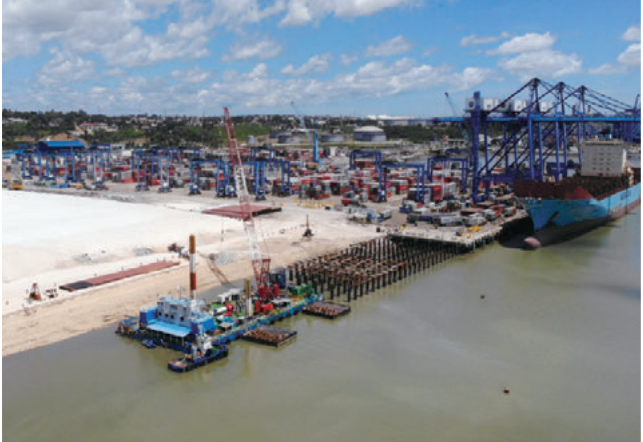
Steel pipe piles were installed by our multipurpose crane vessel. With the use of a pile keeper, 50-meter-long piles were driven in the precise position.
