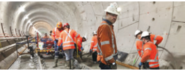
Sydney Metro project in Australia
