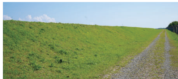
An approximately 600-meter-long embankment constructed within the airport premises
