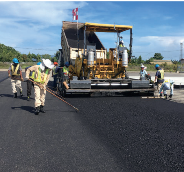
Asphalt concrete paving work for apron expansion
