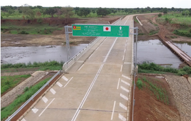
Construction of two bridges, Kara and Koumongou where our product was used in the concrete pavement
