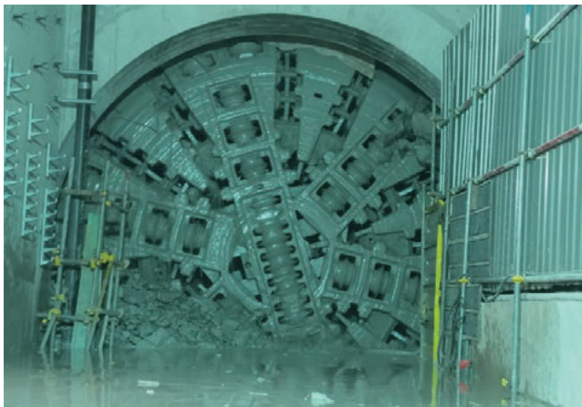
The TBM that successfully broke through after tunneling through complex ground conditions consisting of hard granite and soft soil
