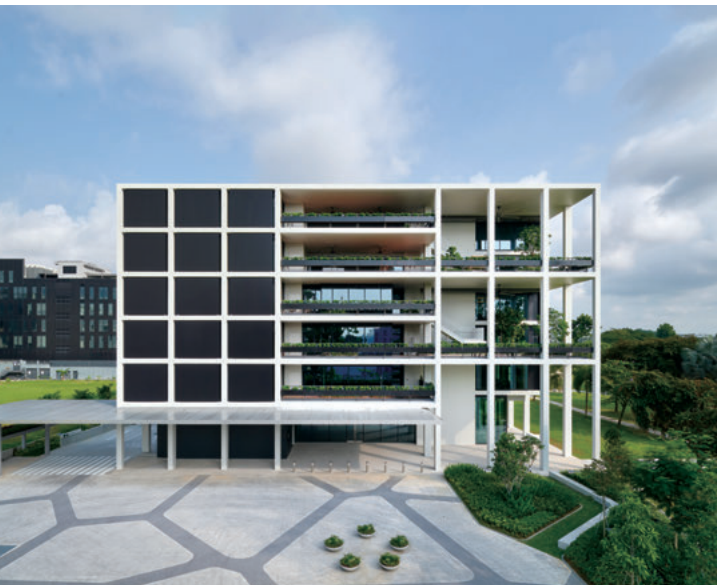
Living Lab Exposed structural frame with thorough skelton-infill concept
