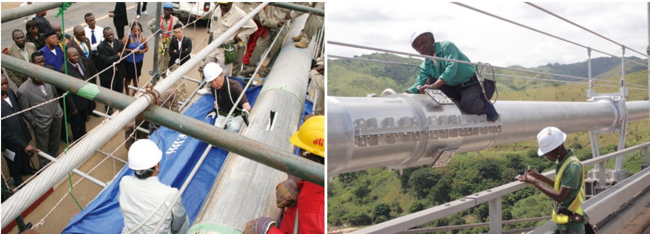
The explanation of the inspection status of the inside of the cable to the attendees of a seminar held at the site (planned by MADIATA to make the government, academia and the private sector aware of the importance of the maintenance and management) Humidity measurement work at the exhaust unit at the center of the bridge
