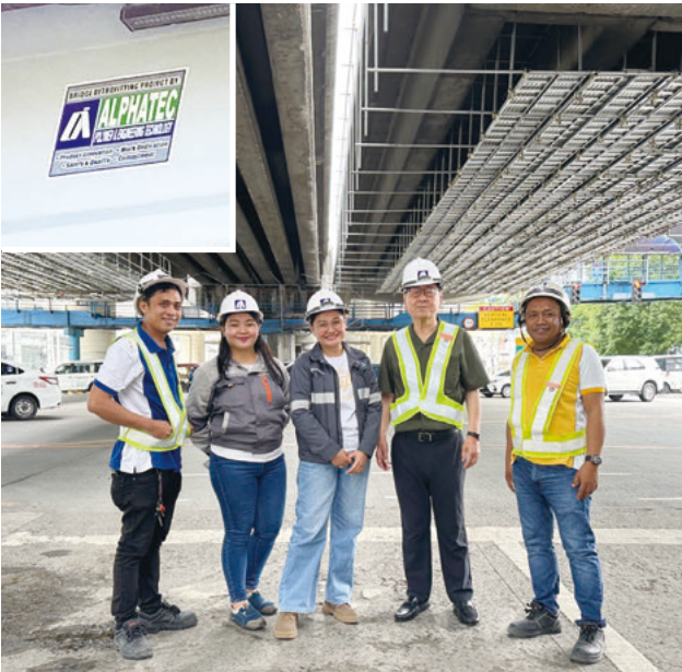
Cracks in deteriorated bridges in Manila were repaired with penetrating epoxy repair material ALPHATEC 380 and then reinforced with carbon fiber.
