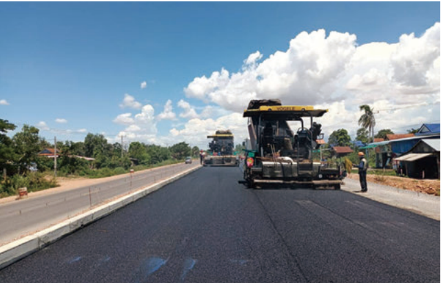
This is the first large-scale pavement project that IKEE LTD. was involved in overseas. (The pavement condition of the 44.1km, National Road No. 5 improvement project in Cambodia.)
