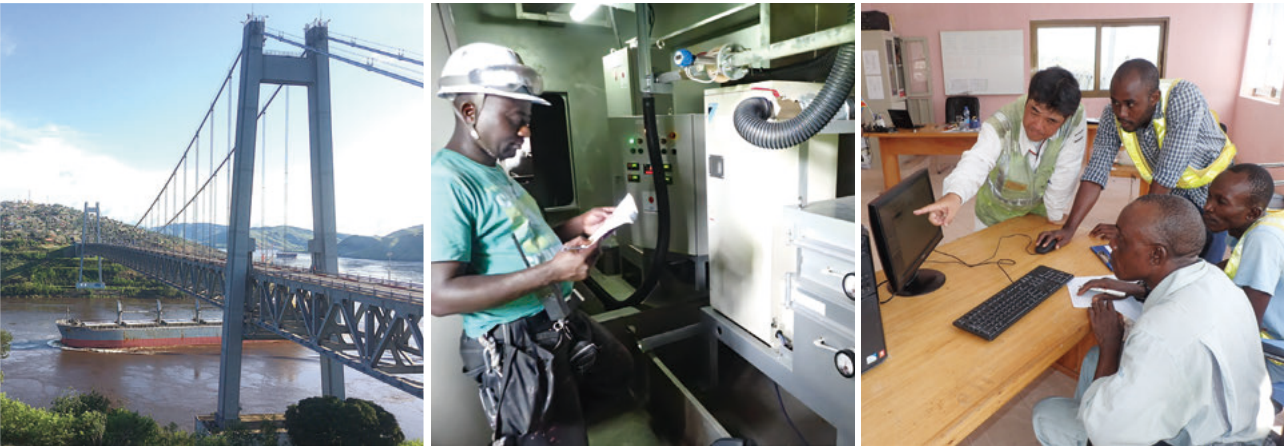
The Matadi Bridge and a cargo ship sailing 150km up the Congo River from the Atlantic Ocean The dehumidification system for the cable installed in the main tower The explanation of how to handle the dehumidifying system for the cable by Japanese engineer to young OEBK engineers (Technical transfer)
