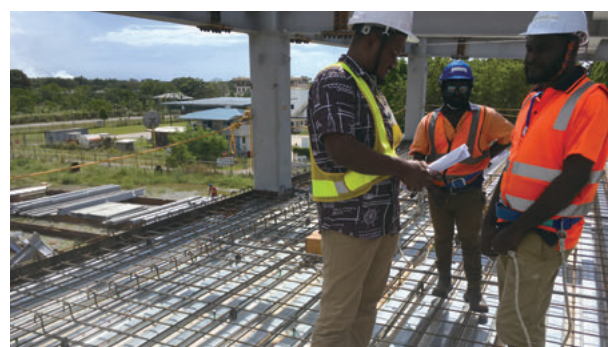
Local engineer employed by Gyros Corporation conducting quality inspections
