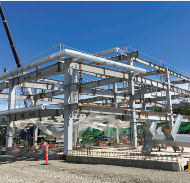
Steel frame erection work for the new international departures terminal building
