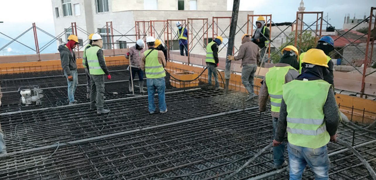
Distribution Reservoir Slab Concrete Placement
