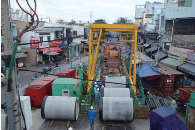
Pipe jacking construction site view. (Total view of departure construction site)
