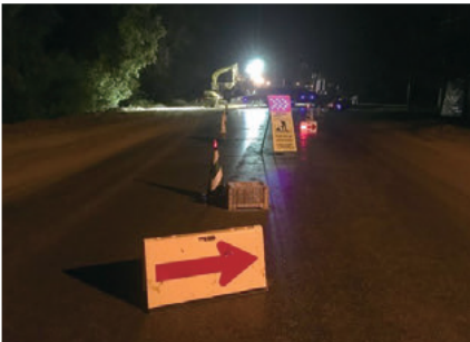
Safety Measures for Nighttime Pipeline Construction Areas
