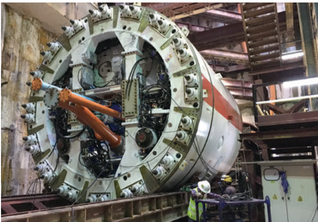
Assembly of a slurry-type Tunnel Boring Machine
