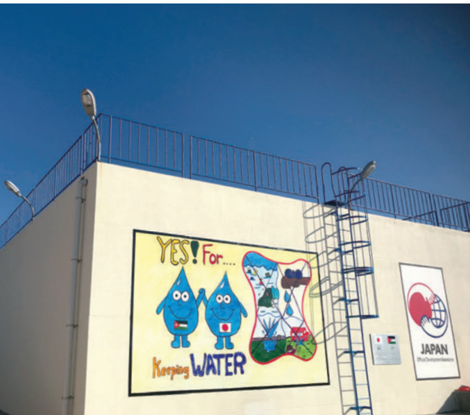
Overview of Distribution Reservoir Two reservoirs were constructed for a gravity-flow system. Among them, a RC reservoir with a capacity of 900m³ was built on elevated ground. and also, Water conservation posters collected from nearby elementary schools were painted on its walls.
