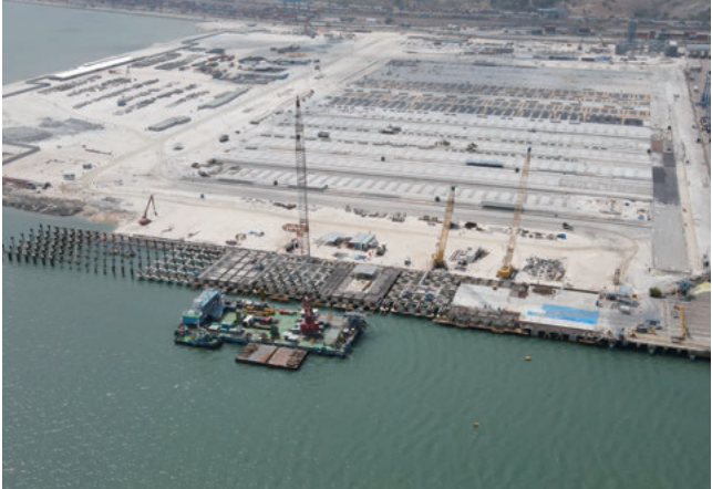
Panoramic view of the project at its peak. Approximately 2,000 workers engaged in marin and land civil work, building and utility works.
