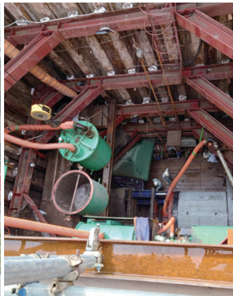
Installation of sewer pipe line at 10 meter underground in Ho Chi Minh city. Horizontally pushing RC sewer pipe into the ground using hydraulic jack at the bottom of departure shaft.
