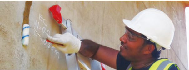
Crack application repair of a bridge with ALPHATEC 380 in Zambia
