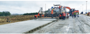
Concrete pavement project in Paraguay
