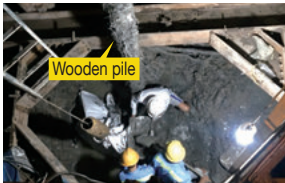
Wooden pile←Pulling out after shaft construction around
