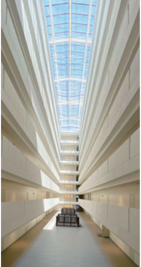
To prevent heat from accumulating in the atrium, double slabs were installed under the second floor level for ventilation, along with a new CFD-simulated natural ventilation system. During the construction period, the atrium was used for material delivery to enable an efficient supply of construction materials. Priority management was exerted with respect to the wall gradient and right angle accuracy of the handrails in the corridor, which significantly influence the appearance of the atrium.
