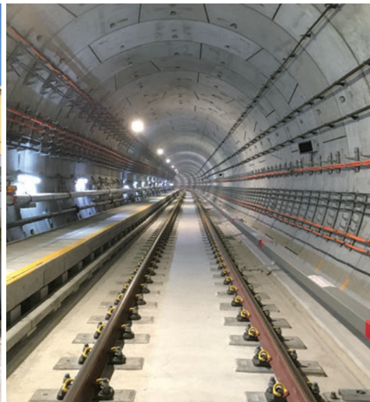
Completed Bored Tunnel
