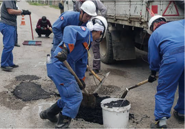
Construction technology transfer of all-weather type pavement repair materials in the Kyrgyz republic. (Using Kyrgyzstan-made pavement repair materials manufactured through the transfer of manufacturing technology)
