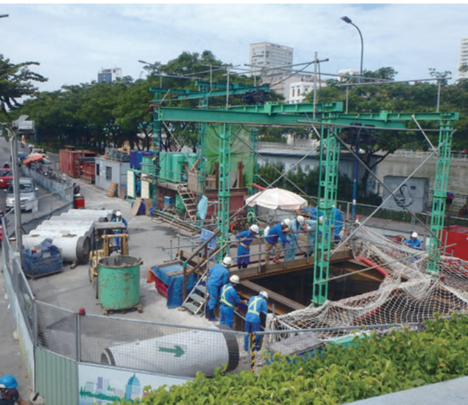
Construction site in the city set up as starting shaft for the first ever large scale sewer system construction in Ho Chi Minh city using pipe jacking construction method.
