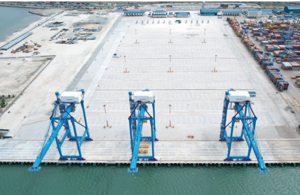
Kenya's first container terminal using reclamation method on soft ground.
