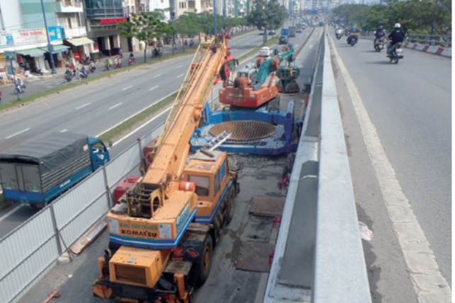
View of shaft construction (Steel casing method: one of the items for changes from original plan)
