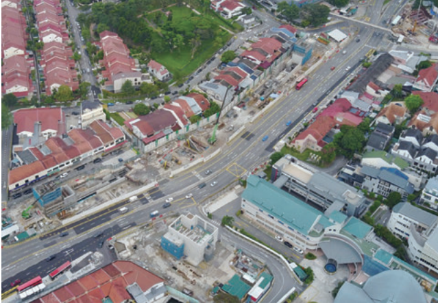
Construction of the Upper Thomson station directly underneath a heavy road using the top-down method in a highly constrained work site
