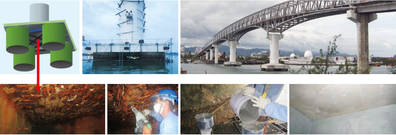
The Mactan-Mandau Bridge in the Philippines, built in 1973, was repaired at low tide with underwater-cured epoxy grout for piers that had deteriorated due to salt damage, without installing steel sheet piles or other materials for closure.
