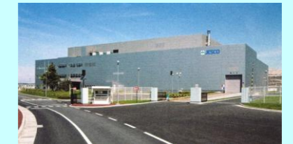
Hokkaido PCB Waste Treatment Facility
