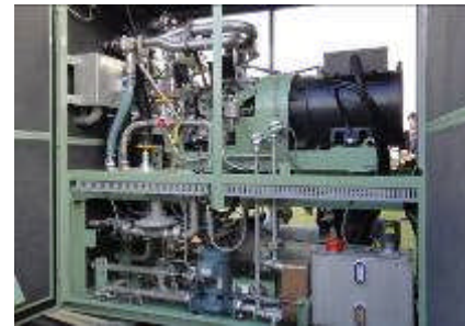
Digestion gas power generation
