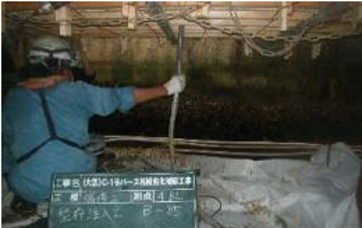
Mortar grouting
