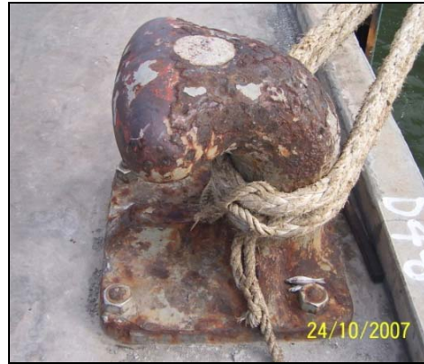
Plate 1.5 : Severe corrosion of bolts, nuts and base plates of bollards
