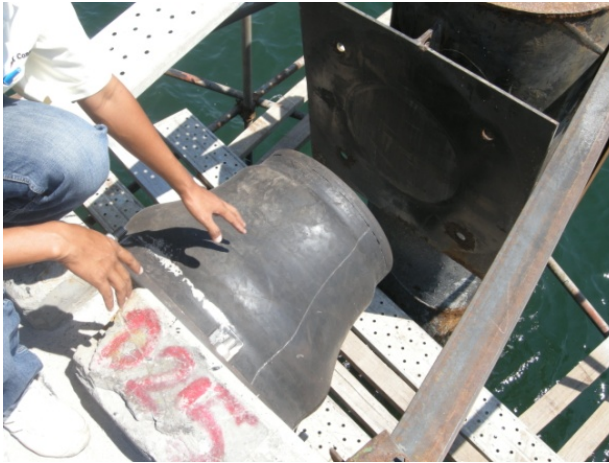
Plate 1.8 : Installation of new rubber fender to replace the deformed fender.
