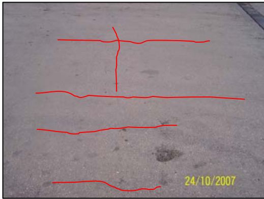
Plate 1.2 : Longitudinal & transverse cracks (red lines drawn alongside the cracks to highlight them)
