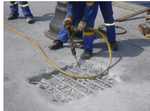
Plate 1.14 : Removal of defective concrete prior to repair.
