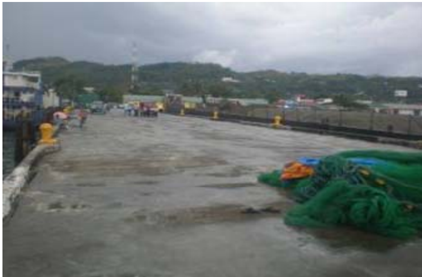
Figure 1.2 Deck view of R.C. Pier - 2
