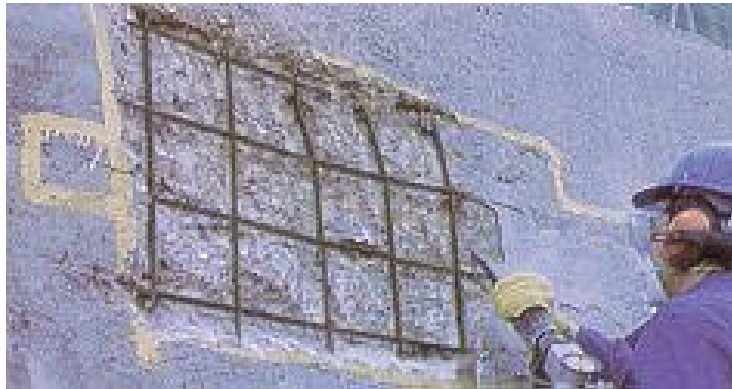
Plate 4.10 : Breaking out of defective concrete
