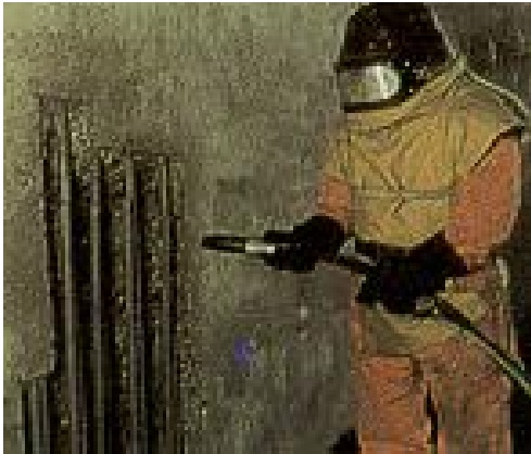
Plate 4.12 : Grit Blasting the Steel
