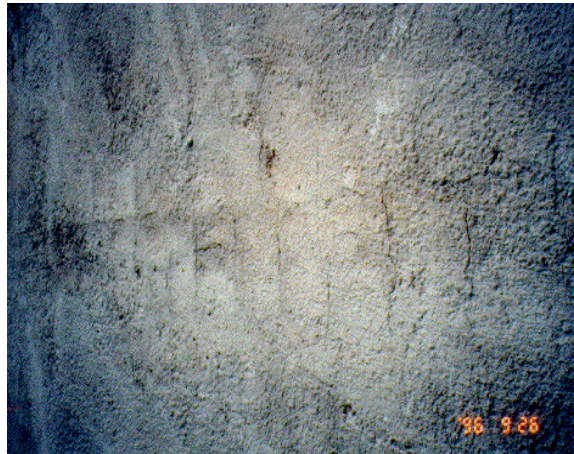
Plate 3.4 : Cracks in floor slab following line of reinforcement.
