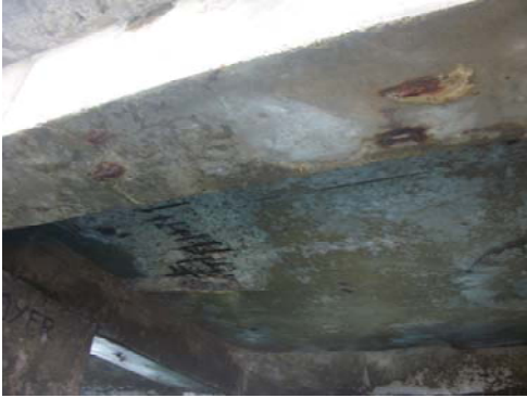
Picture 1.1 Condition of bottom deck on wharf and trestle (the Waren port)
