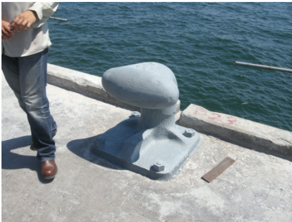
Plate 1.11 : Repaired corroded steel bollard and applied with protective coating.
