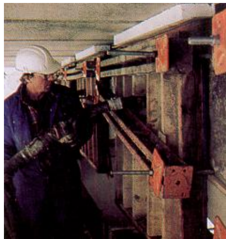
Plate 4.17 : Pumping to formwork
