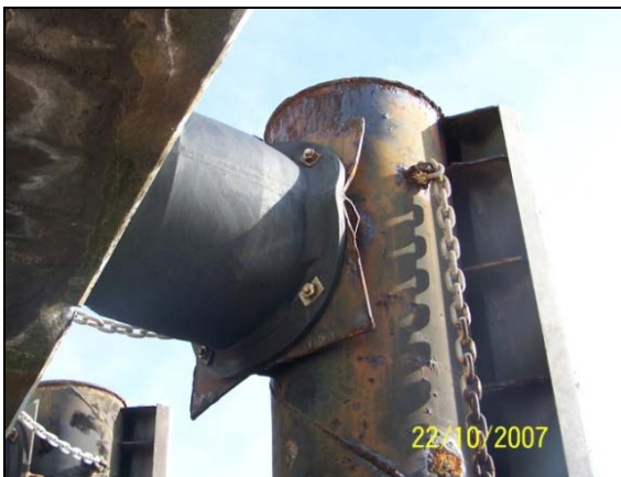
Plate 1.4 : Deformed rubber and corrosion of the fenders
