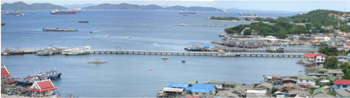
Figure 1.2 View of Sri Chang jetty
