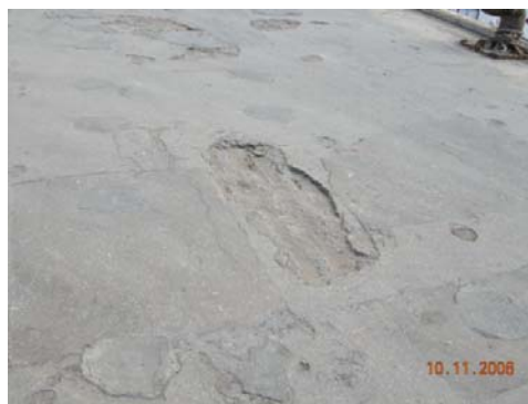
Plate 4.6 : Minor delamination in deck slab will deteriorate further if no action is taken and therefore should be patch repaired immediately.
