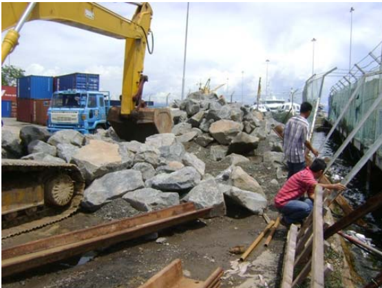
Plate 1.17 : Work for revetment of damaged slope protection.
