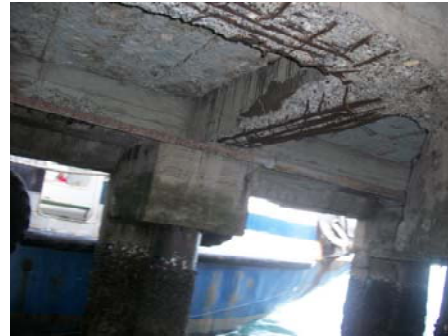
Picture 1.1 Condition of bottom deck on wharf and trestle (the Waren port)
