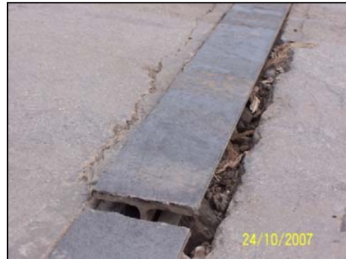
Plate 1.6 : Damaged joint leaving a gap and leakage
