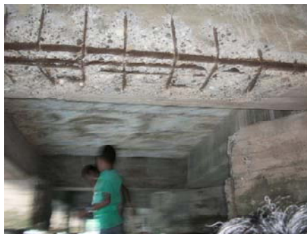
Picture 1.2 Condition of beam on Waren port
