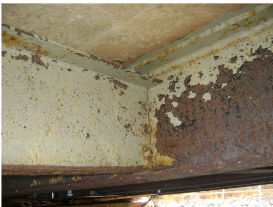
Plate 4.20 : Paint deterioration and mild surface corrosion of steel beam can lead to widespread corrosion if left unattended.
