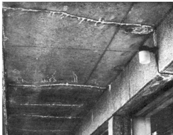
Plate 3.5 : Transverse cracks in slab.
