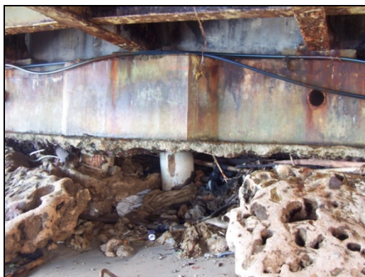
Plate 4.4 : Damaged rubble pitching need restoration before condition worsen.
