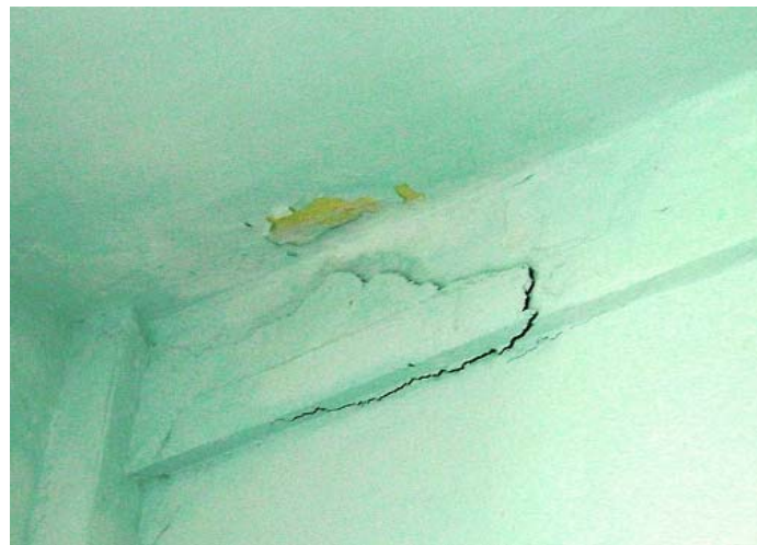
Plate 3.2 : Delamination of concrete due to expansion of corroded reinforcement.
