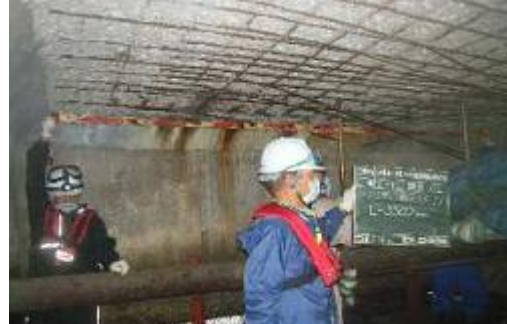
Removing cover concrete
