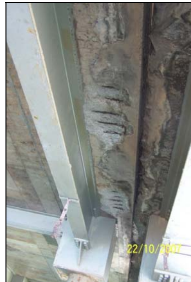
Plate 1.7 : Severe spalling of concrete with exposed reinforcement bar
