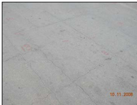
Plate 4.5 : Cracks in concrete deck allow water to seep through them and wet the underside of the wharf deck. They can be repaired by sealing with epoxy resin.
