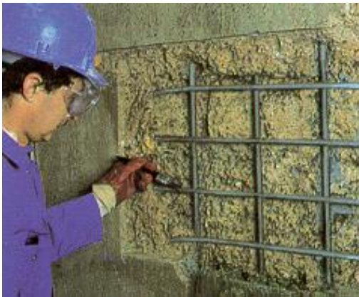
Plate 4.13 : Priming Steel
