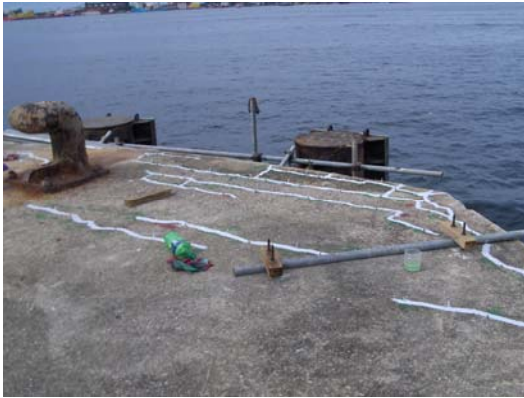
Plate 4.7 : Crack Injection repair at the dolphin of Kuantan Port Wharf
