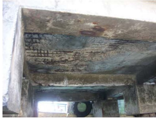
Picture 1.1 Condition of bottom deck on wharf and trestle (the Waren port)
