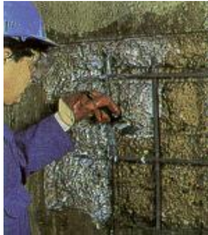
Plate 4.15 : Applying bonding aid
