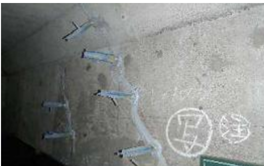
Crack injection
