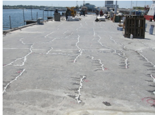
Plate 1.13 : Sealed cracks after injection with epoxy resin.
