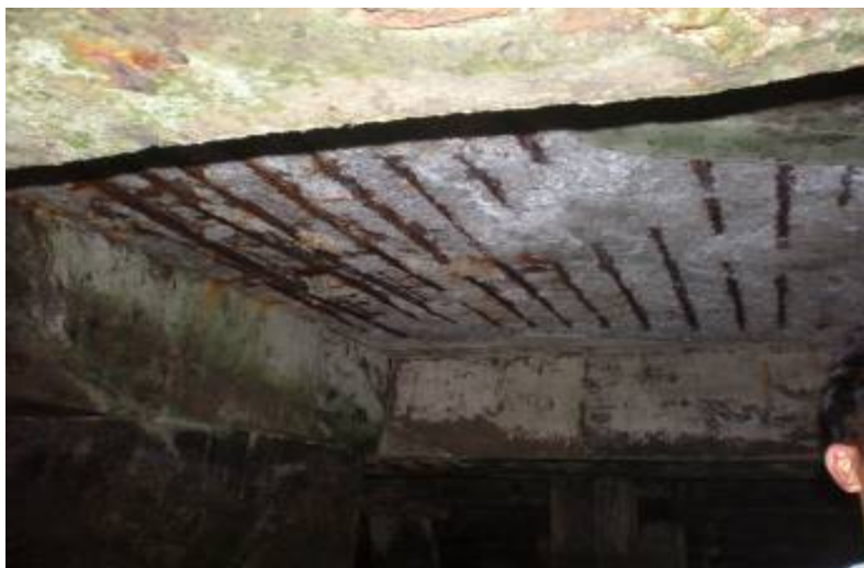
Figure 1.5 Underdeck view of portion of R.C. Pier - 2 showing damaged r.c. deck
