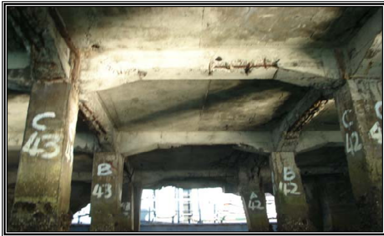
Figure 1.4 Underdeck view of portion of R.C. Pier - 2 showing damaged r.c. beams
