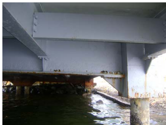
Plate 4.21 : Steel Beam appearance after coating
