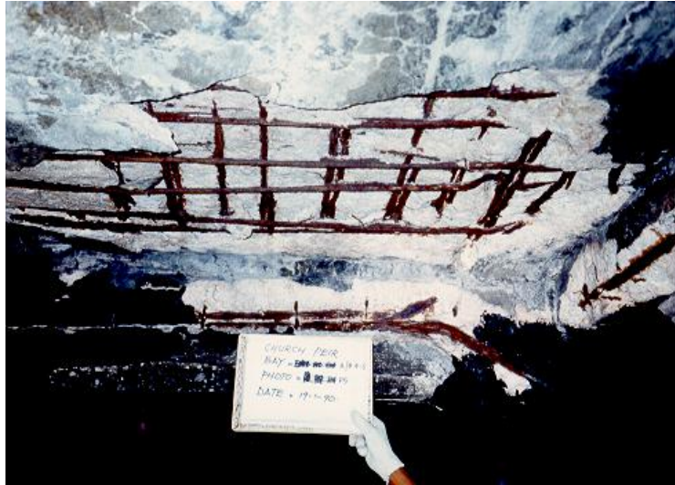
Plate 3.1 : Spalling of concrete due to expansion of corroded reinforcement.
