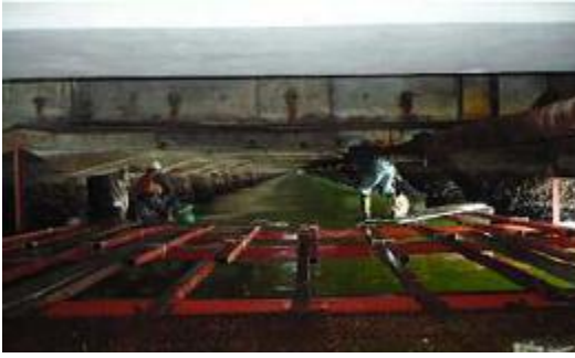
Setting of scaffold
