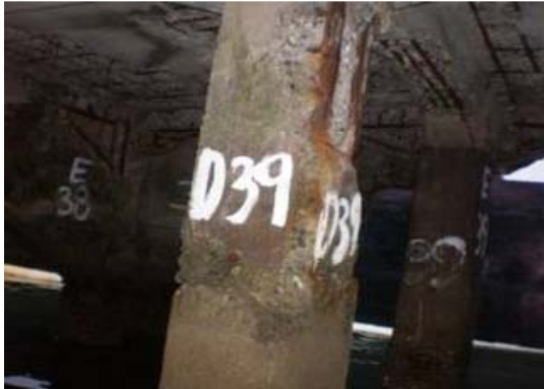
Figure 1.6 Underdeck view of portion of R.C. Pier - 2 showing damaged r.c. piles
