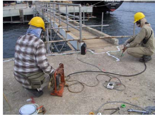
Plate 4.8 : Crack injection repair being carried
