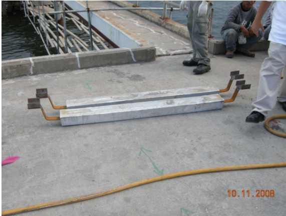
Plate 1.16 : Sacrificial anodes for installation of cathodic protection system to fender piles.
