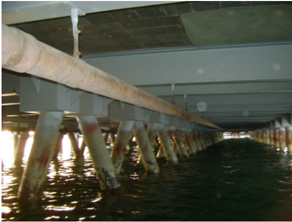
Plate 1.10 : Repaired and painted corroded steel beams and pile caps with protective coating system.
