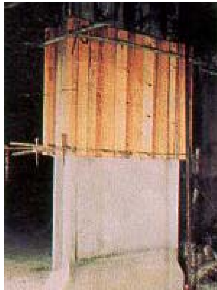
Plate 4.16 : Grout-tight formwork
