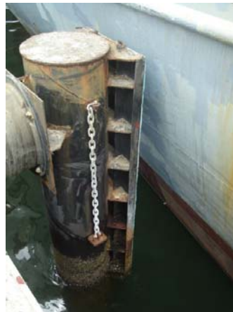
Plate 4.3 : Detached shear chain of the fender should be reinstated
