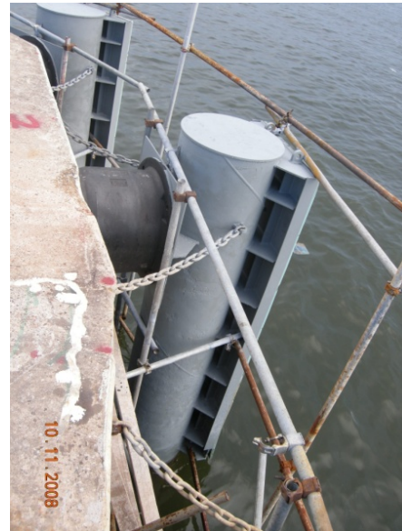
Plate 1.9 : Completed installation of new rubber fender and coating of fender pile.
