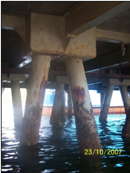
Plate 1.3 : Substantial corrosion of steel piles
