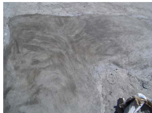
Plate 1.15 : Completed repair of defective/spalled concrete
