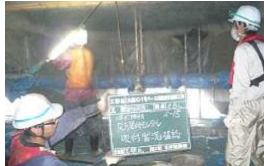
Mortar spraying
