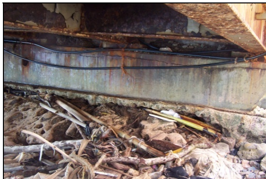
Plate 4.1 : Debris retains dampness and should be removed to avoid corrosion of steel beams.
