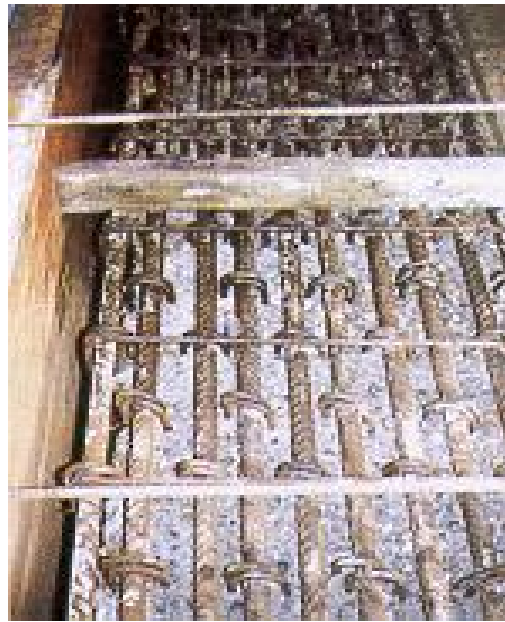
Plate 4.19 : Congested area of rebar
