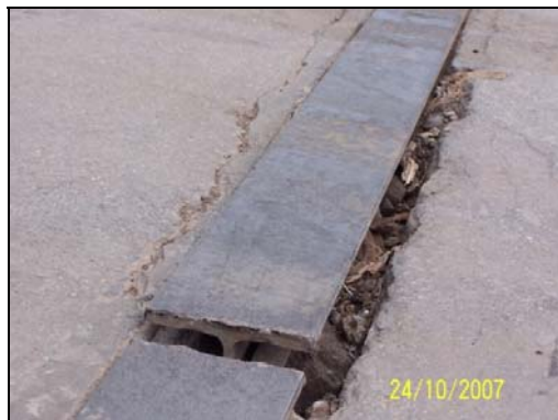
Plate 4.2 : Damaged expansion joint in need of replacement
