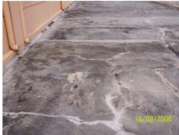
Plate 3.3 : Random patterned cracks in floor slab.
