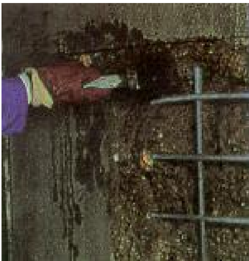
Plate 4.14 : Wetting of substrate
