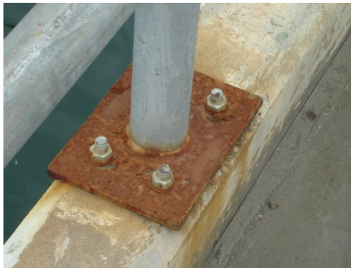
Plate 4.22 : Bolts and nuts should be tightened
