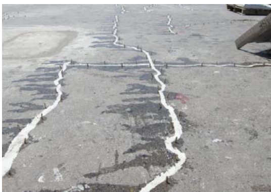
Plate 1.12 : Installation of injection ports in preparation for epoxy injection.
