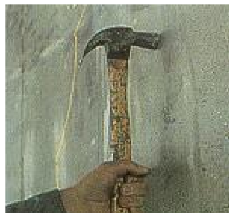
Plate 2.4 : Sounding (Hammer) Test
