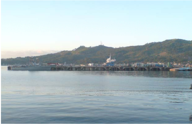
Figure 1.3 Longitudinal view of R.C. Pier – 2
