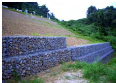
< 盛土のり尻補強 >
