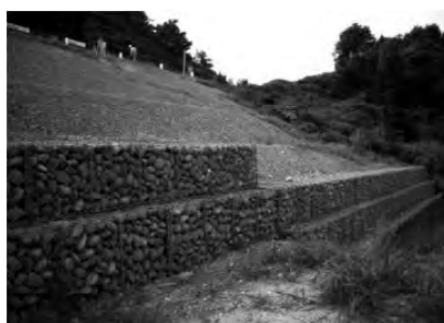
< 盛土のり尻補強 >
