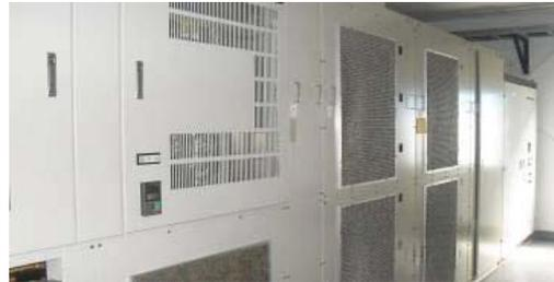
*380-600V & 3.3 kV - 6.6 kV Motor Control Center with Variable Spee Drive*
