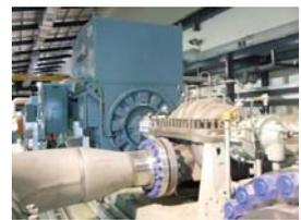
High pressure seawater supply pump for RO desalination in Australia
