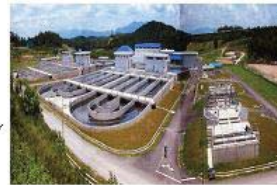
WWTP in Malaysia (59,000 m 3 /d)
