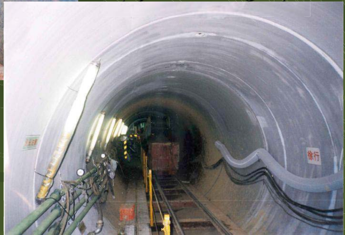
Muck transportation (by muck wagon)
