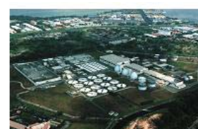
WWTP in Singapore 75,000 m 3 /d
