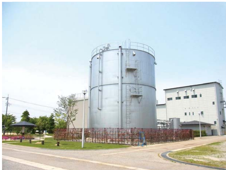
Delivered in 2011 [ 80m 3 /day ]
