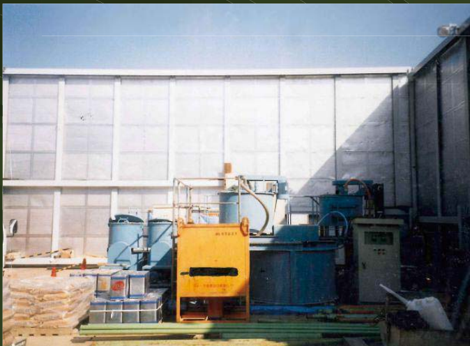
Lubrication & Backfill grouting Plant
