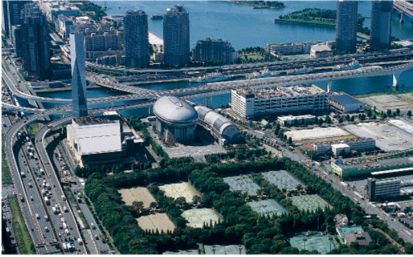
Ariake sewage treatment plant (Tokyo, 300,000 m 3 /day, 1994)
