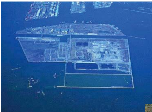
Landfill Leachate treatment (Tokyo, Total 20,500 m 3 /d, 1979, 1986, 2000)
