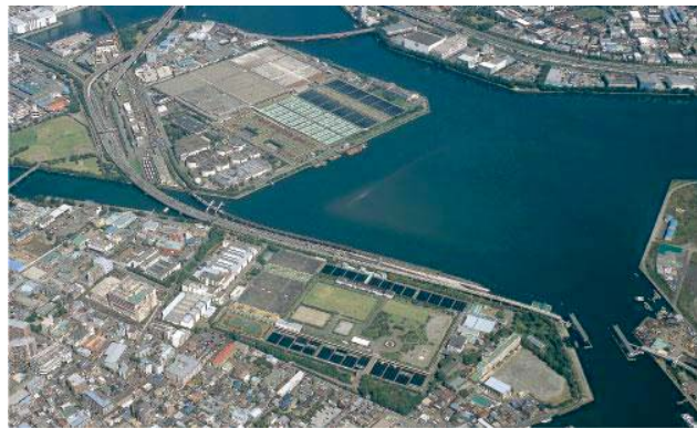
Morigasaki sewage treatment plant (Tokyo, 1,5400,000 m 3 /day, 1966)
