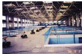
WWTP in China (260,000 m 3 /d)
