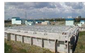
WWTP in Vietnam (141,000 m 3 /d)
