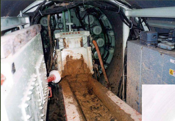
Muck discharge (behind the shield)
