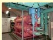
Heat exchange system using raw sewage
