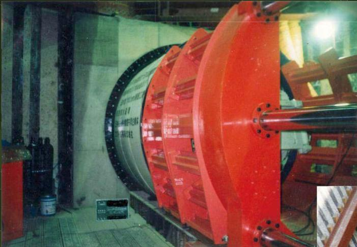
Jacking pipe is dropped into the shaft and placed on the support rails.
