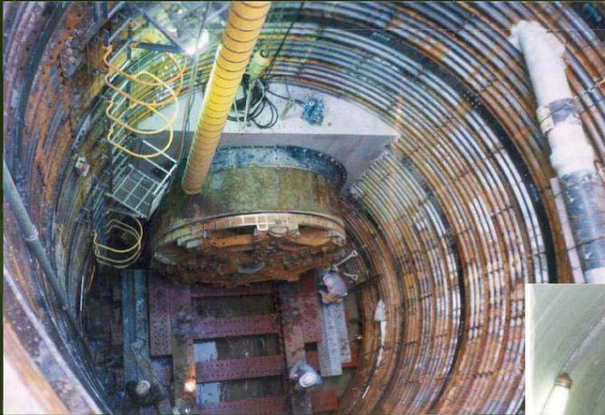
After reception, backfill grouting is carried out
