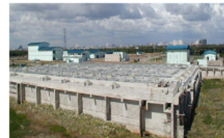
WWTP in Vietnam (141,000 m 3 /d)
