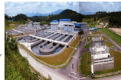
WWTP in Malaysia (59,000 m 3 /d)
