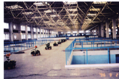
WWTP in China (260,000 m 3 /d)
