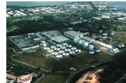
WWTP in Singapore 75,000 m 3 /d
