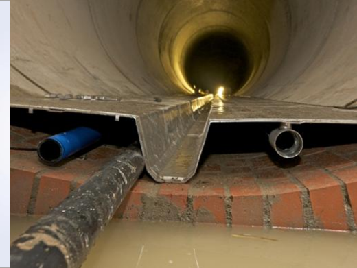
Gutter heat exchanger at the bottom of the sewer
