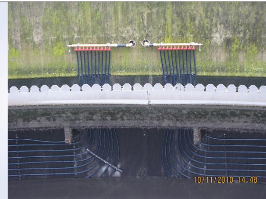
Use of treated wastewater - final clarification
