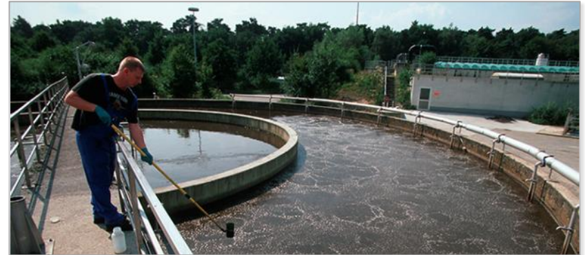
Waste water treatment plant Dorsten-Wulfen
