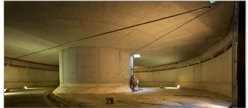
Storm water retention basin Haarbach in Gladbeck
