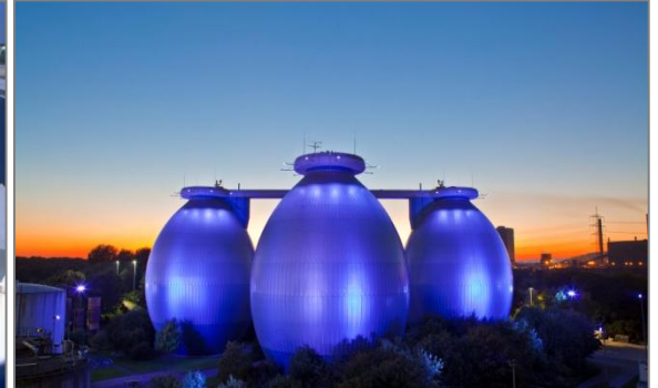
Waste water treatment plant Bottrop
