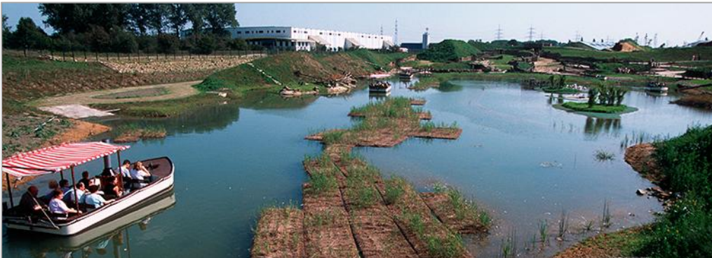
53 Flood water retention basins, 3.8 Mio. m 3 retention volume
