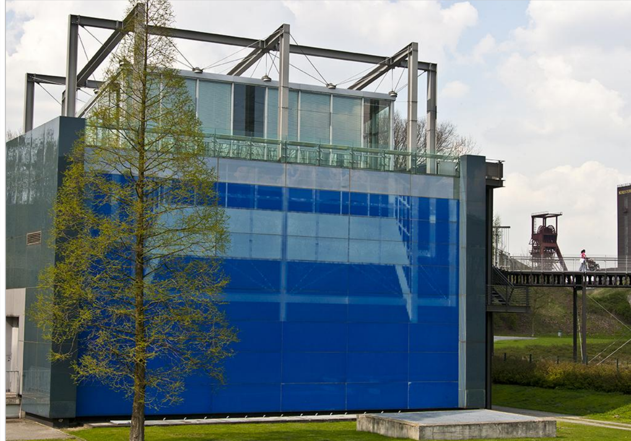
302 Pump stations, 842 km 2 Polder areas
