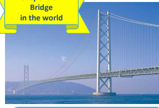
Akashi Kaikyo Bridge Aug.1989~Mar.1998 3,911m Center Span:1,991m
