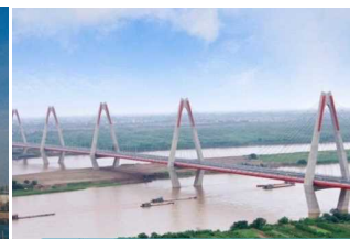
Nhat Tan Bridge Vietnam Oct.2009~Oct,2014 1,500m Center Span:300m x 4
