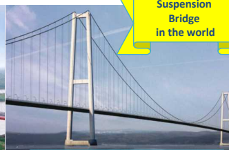
Izmit Bay Crossing Turkey Jan.2013~Feb.2016 Under Construction 2,682m Center Span:1,550m
