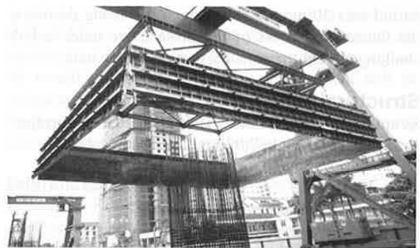
Fig.5 Form of pile cap
