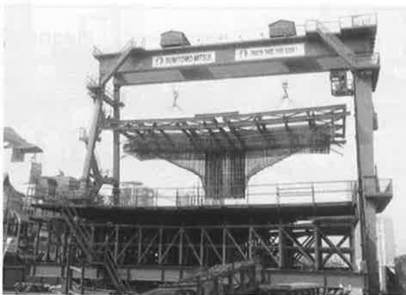
Fig.8 Installation of pre-assembled rebar
