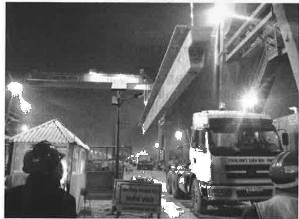
Fig.10 Erection of super-t girder
