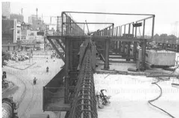
Fig.12 Parapet work by gondola
