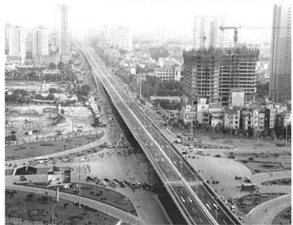
Fig.13 Completion and traffic open
