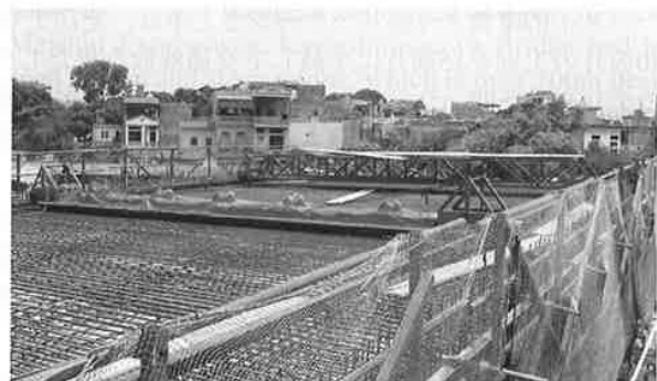
Fig.11 Finishing of slab-surface concrete
