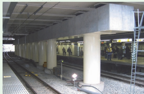
Replaced bridge in 2012
