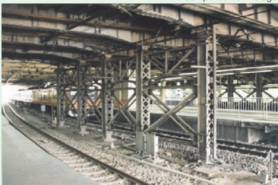
Old bridge built in 1925
