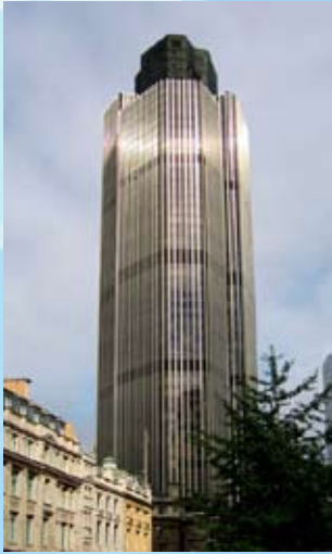
Tower 42, London's Tallest Building Photograph © Andrew Dunn
