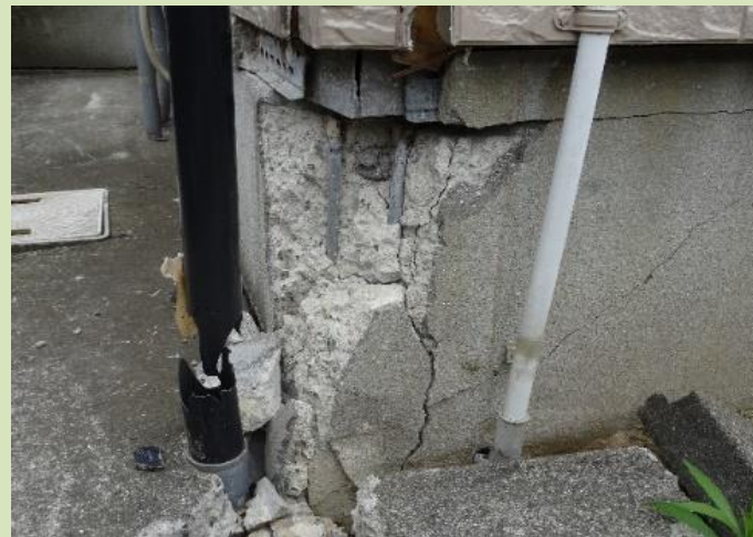
[出隅部の被害]
