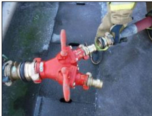
Step 2 Attach the 40 mm fire hose to the Y gate valve.
