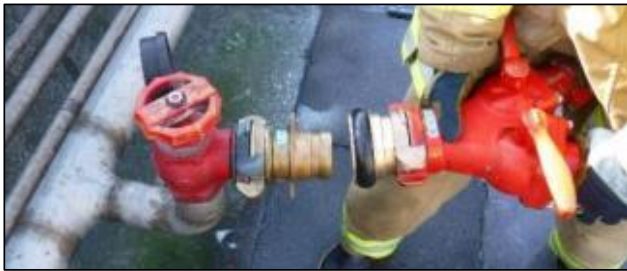
Step 1 Connect the Y gate valve to the hydrant.
