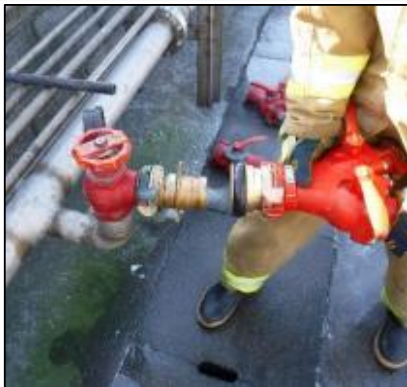
Step 1 Attach the Y gate valve to the 65 mm hydrant.
