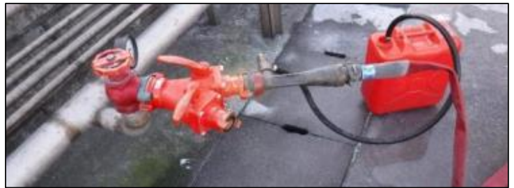
Step 2 Connect the line proportioner of the portable foam applicator to the Y gate valve.
