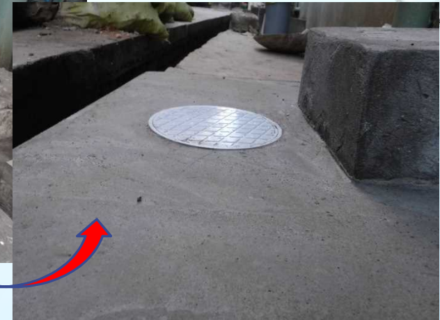
Pilot project on improvement of old sewerage system
