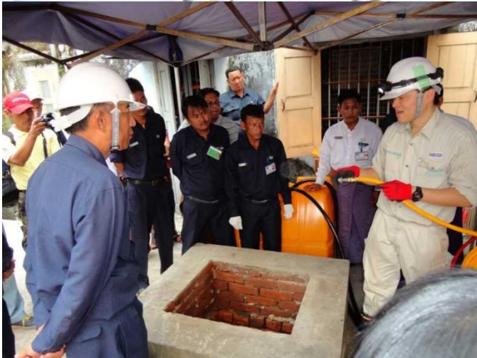
The training of maintenance of sewer
