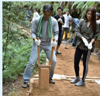
Figure 1-3-4 Repairing the Kumano Kodo
