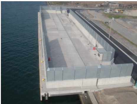
(Guard-fenced, tire-washing, and water-collecting facility)
