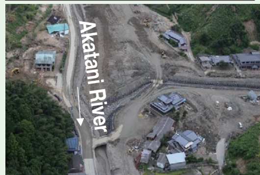
Emergency countermeasures completed
