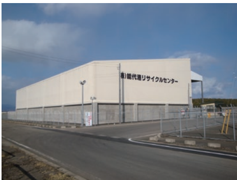
(Storage facilities for contaminated soil, etc.)
