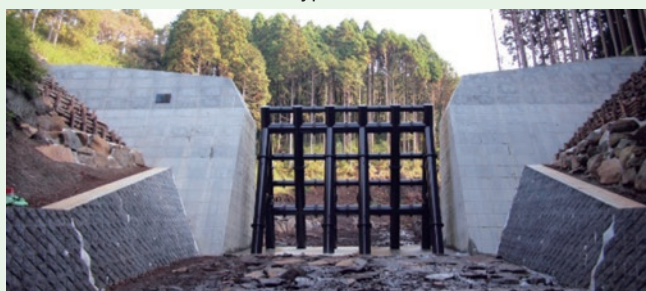
Open-type Sabo dam
