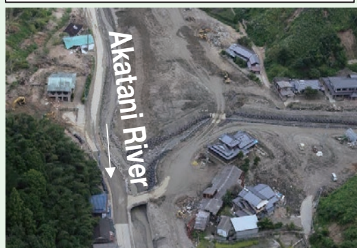
Emergency countermeasures completed
