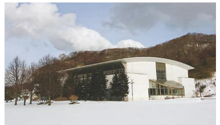
Municipal swimming pool equipped with household fuel cells
