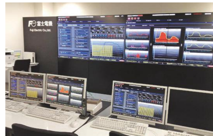
The district's community energy management system
