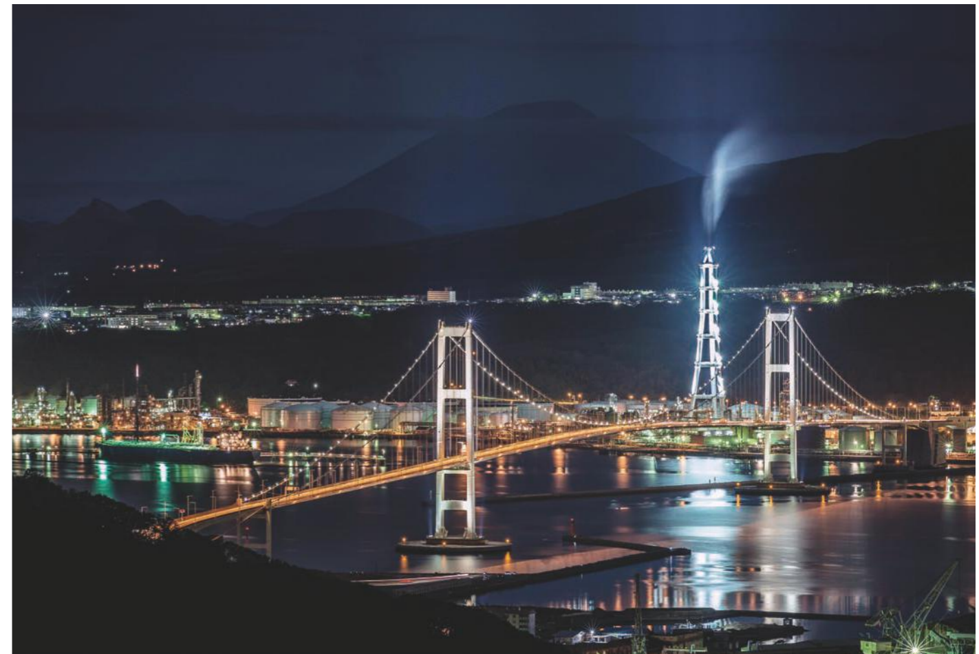
Illumination of Hakucho Bridge uses wind-powered LED lights
