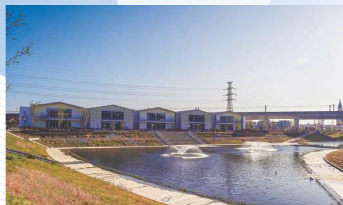
Retention basin integrated into park space
