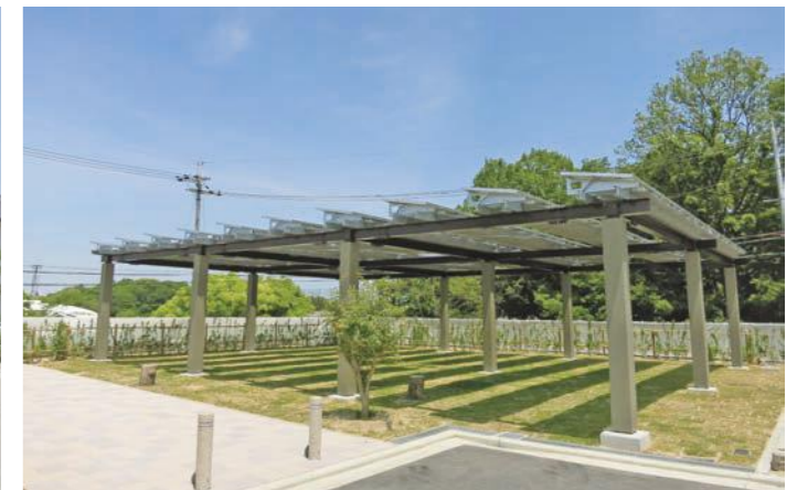
Solar energy system on shared facility
