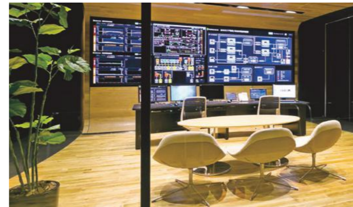
Energy management system
