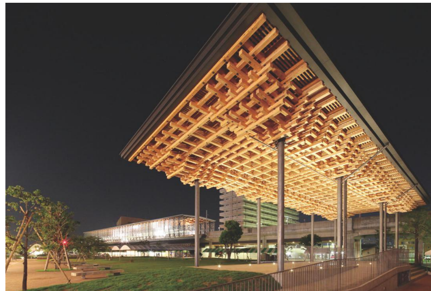
The outdoor stage is built from plentiful local cedar
