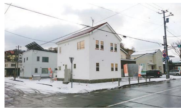
Residential area with fuel cell-equipped homes
