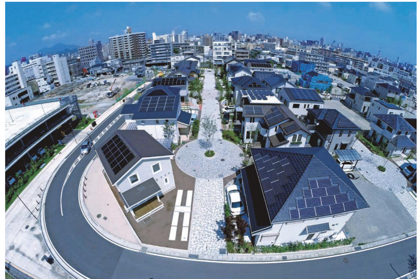
Solar panels installed on houses
