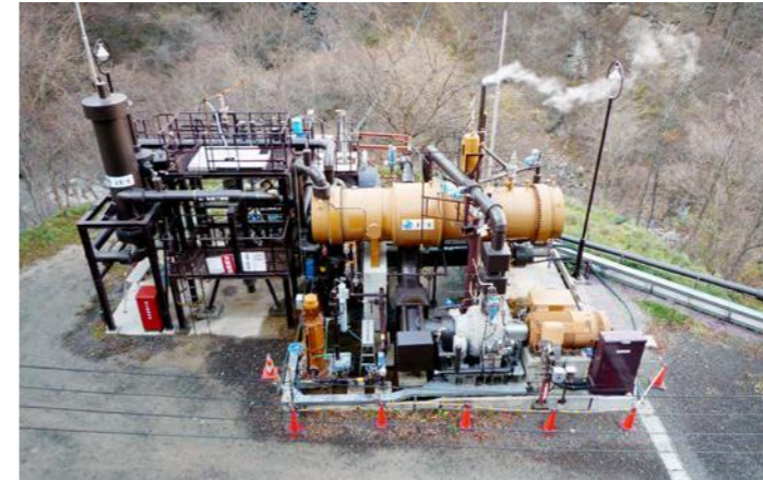
A binary cycle geothermal power plant is a focus of the town plan
