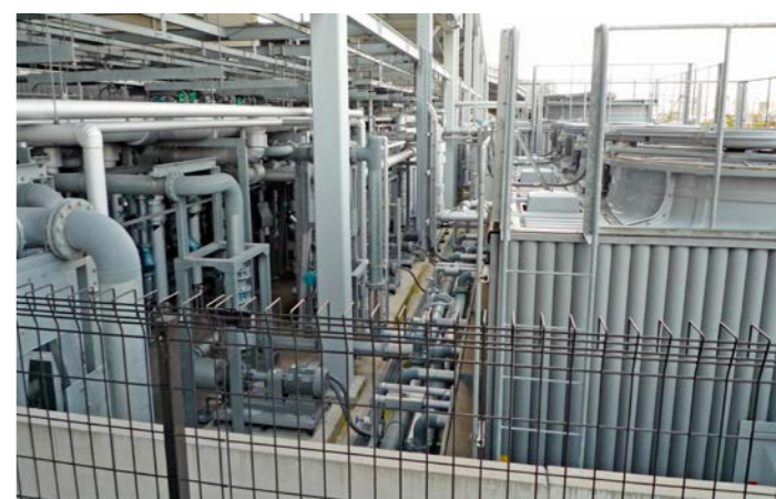
System harvests heat from reclaimed wastewater
