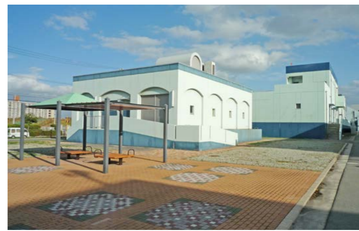
Water supply system at Sambo Water Recycling Center
