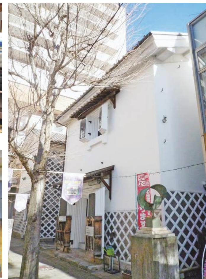
Renovated warehouse is used as management company office
