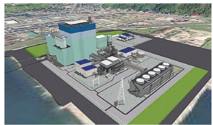
Biomass power generation plant fueled by palm kernel shells is planned to start operation in 2020 (Photo courtesy of Muroran Biomass Power Generation G.K)
