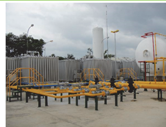
LPG Supply System 50t Tank 1,500 kg/h Air-heating Vaporizer
