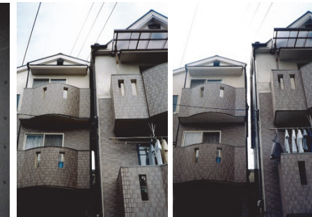
General housing - Before/After releveling
