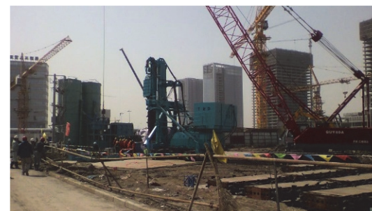
Tianjin, China Diaphragm wall construction
