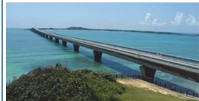
Ikema Bridge Prefecture : Okinawa Year of completion : 1992 Bridge type : PC continuous box girder Products : Viscous dampers with Al-Mg thermal spraying
