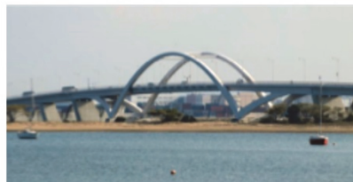
Uminonakamichi Bridge Prefecture : Fukuoka Year of completion : 2014 Bridge type : Arch Products : Bridge bearings with Al-Mg thermal spraying
