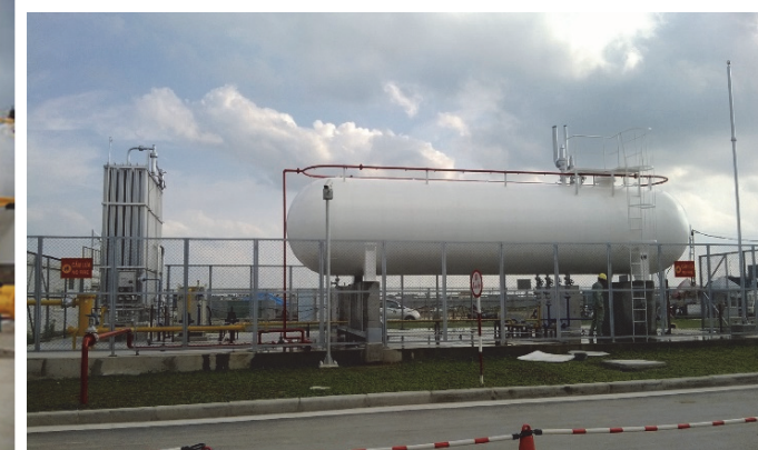
LPG Supply System 25t Tank, Air-heating & Electric Vaporizer
