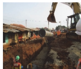
Installing ductile iron pipes (Completed in 2017)
