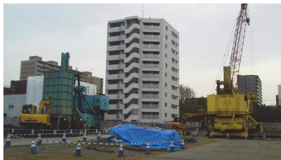
Diaphragm wall construction
