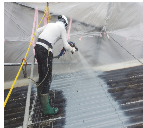
Slate roof sprayed with Polyurea
