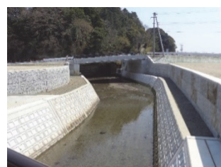
Riverbank retaining wall
