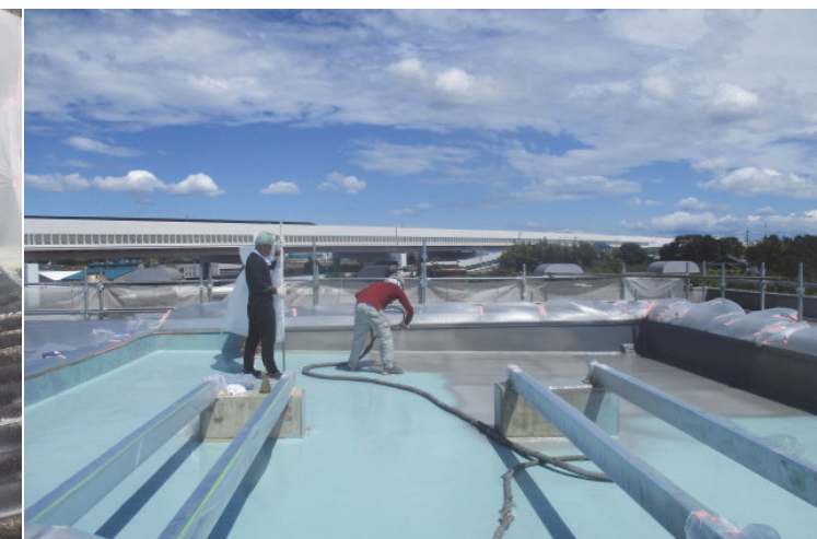
Waterproof rooftop sprayed with Urethane
