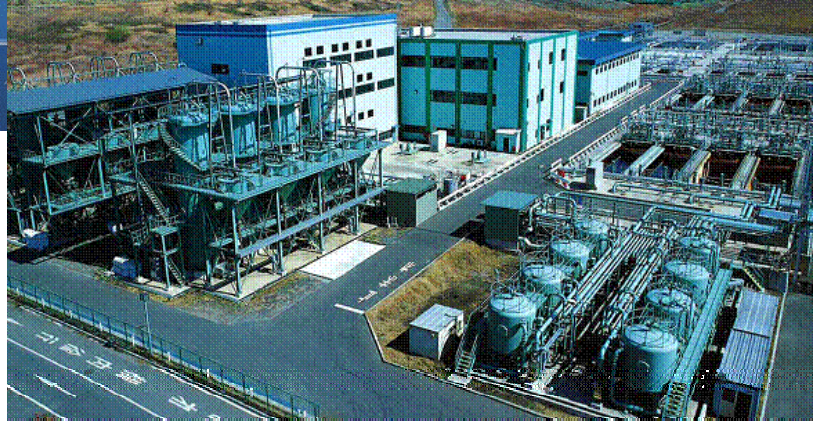
Leachate Treatment in Central Breakwater Landfill Site (20,500 m 3 /d)
