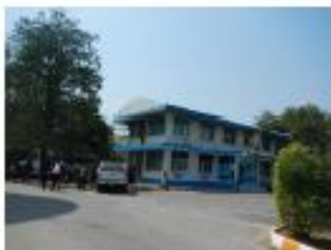
Bangkhla Waterworks 外観
