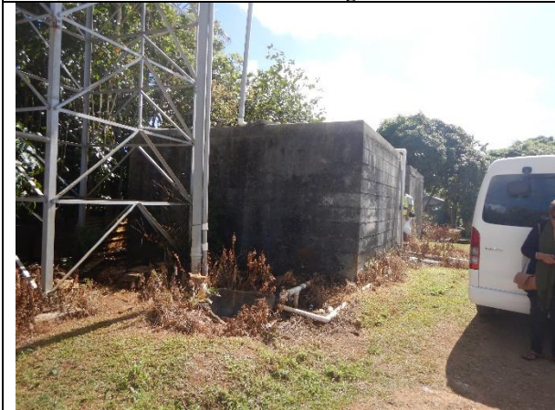
Photo-27: Existing reservoir for Leimatua village water supply, Vava'u Island. Existing reservoir for village water supply in Leimatua. On-site measurements showed a good electrical conductivity of 665 \mu\text{S}/\text{cm} and a residual chlorine concentration of 0.2 mg/l.
