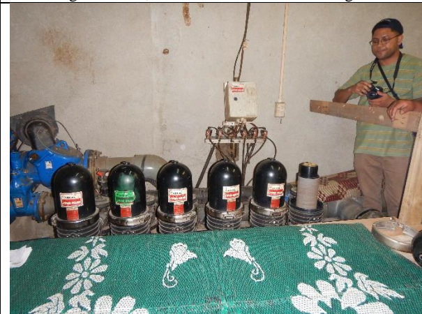
Photo-3: Failed membrane filtration system, Eua Island.
