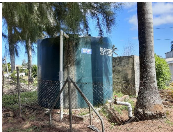
Photo-8: Pressure reducing tank, Eua Island.
