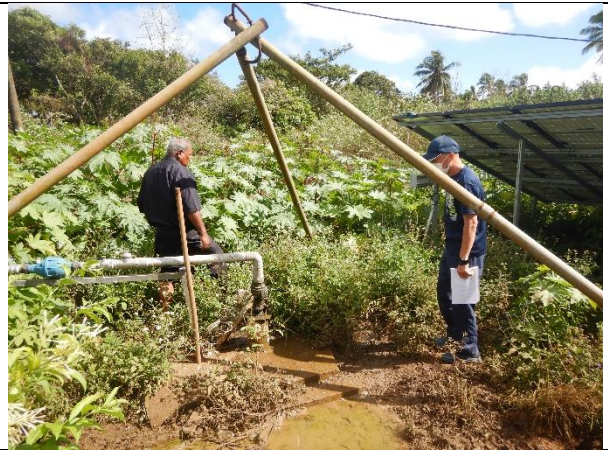
Photo-26: Leimatua village intake pump, Vava'u Island. Solar-powered intake pumps for village water supply in Leimatua. Installed with grant assistance for grassroots human security by Japan. The electrical conductivity of 874 \mu\text{S}/\text{cm} (August 2022).
