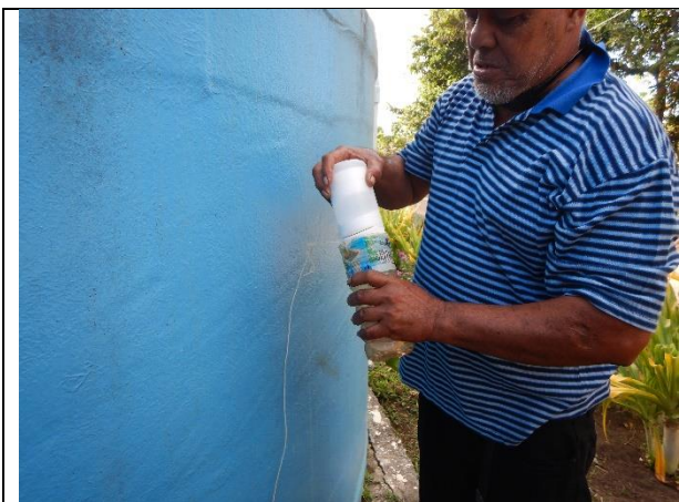
Photo-19: Chlorination with hypochlorite tablets (Lifuka Island).
