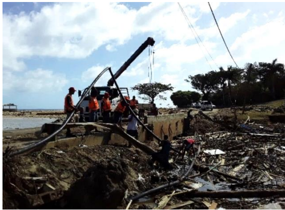
Distribution pipes damaged by the tsunami ('Eua)
