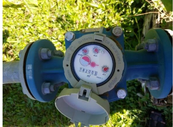
Photo 2.5 Broken Flow Meter
