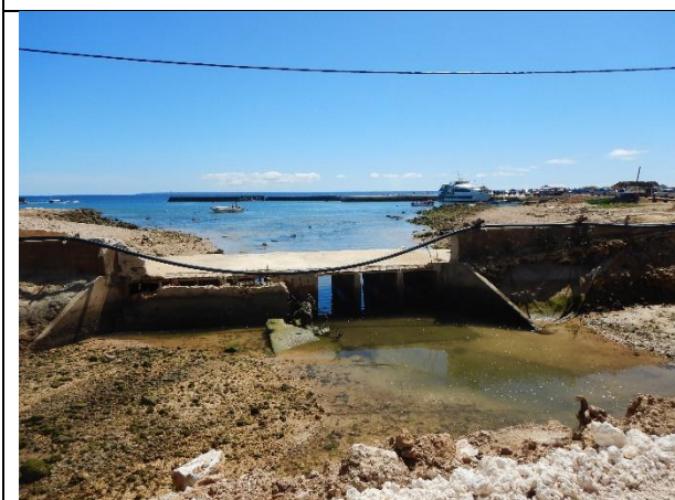
Photo-9: Water distribution pipes damaged by the tsunami, Eua Island.
