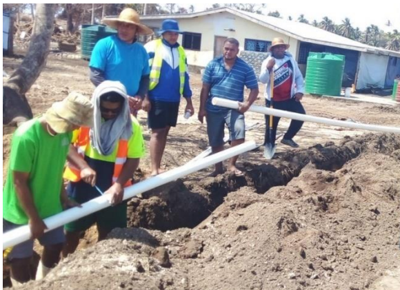
Repairing of distribution main damaged by the tsunami (Tongatapu)
