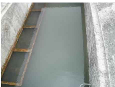
High turbid raw water after rainfall (sedimentation tank receiving chamber)
