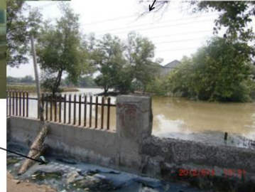
Wall to prevent over flow of sea water in Muara angke (North Jakarta)
