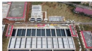
Combined Sewer Overflow system in China
